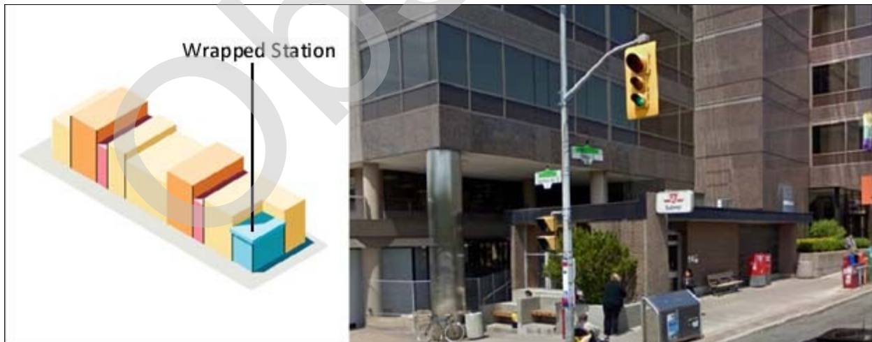
FIGURE B7-3 EXAMPLE OF A WRAPPED STATION
