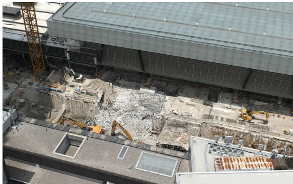
Track slab demolition and site excavation
