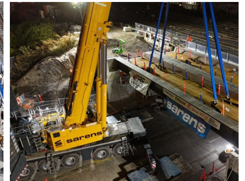
Bridge lifts completed
