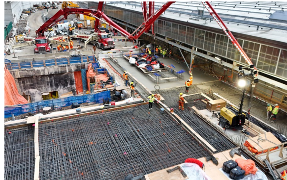
Multiple concrete pours to enable wider platforms and additional rail tracks.
