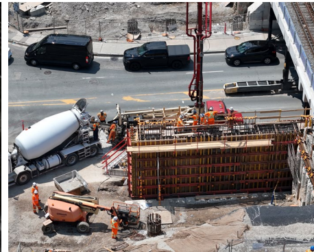
Poured concrete for new abutments at both bridge locations
