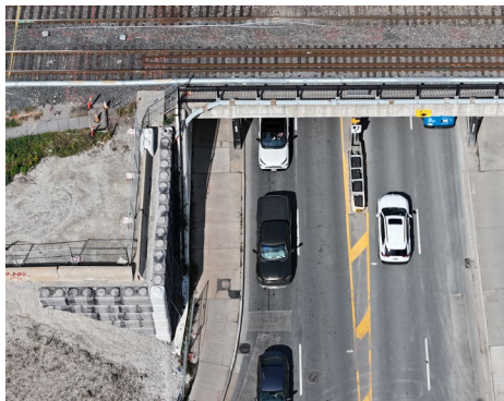
Installed secant wall
