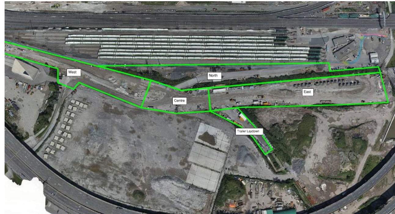
Photo: Wilson Yard Surcharge Zones
