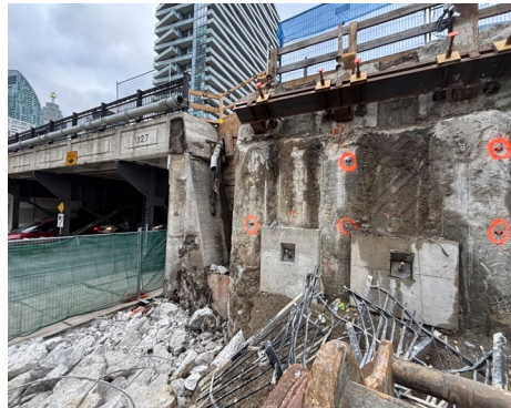
Demolished old wingwall and bridge fascia
