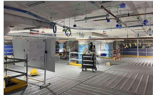
Started the mechanical and electrical fit-out of the newly constructed concourse
