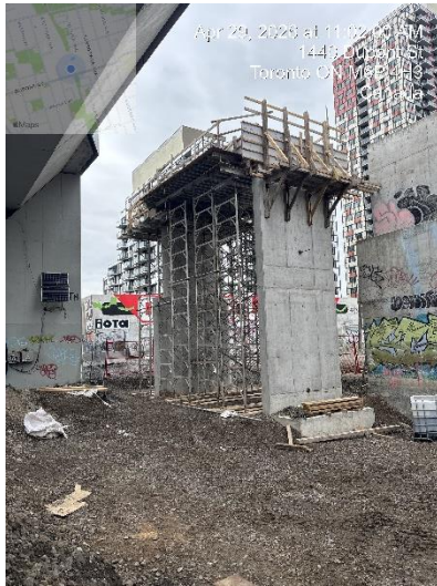
#2 Pedestrian Bridge abutment construction near Dupont St
