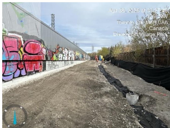
#1 In-corridor works near Davenport Village Park
