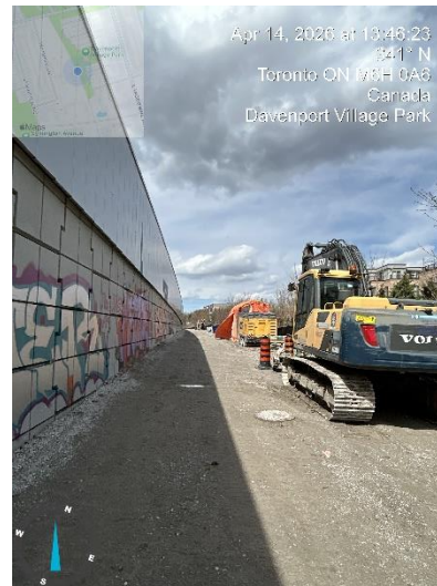
#3 In-corridor works near Davenport Village Park
