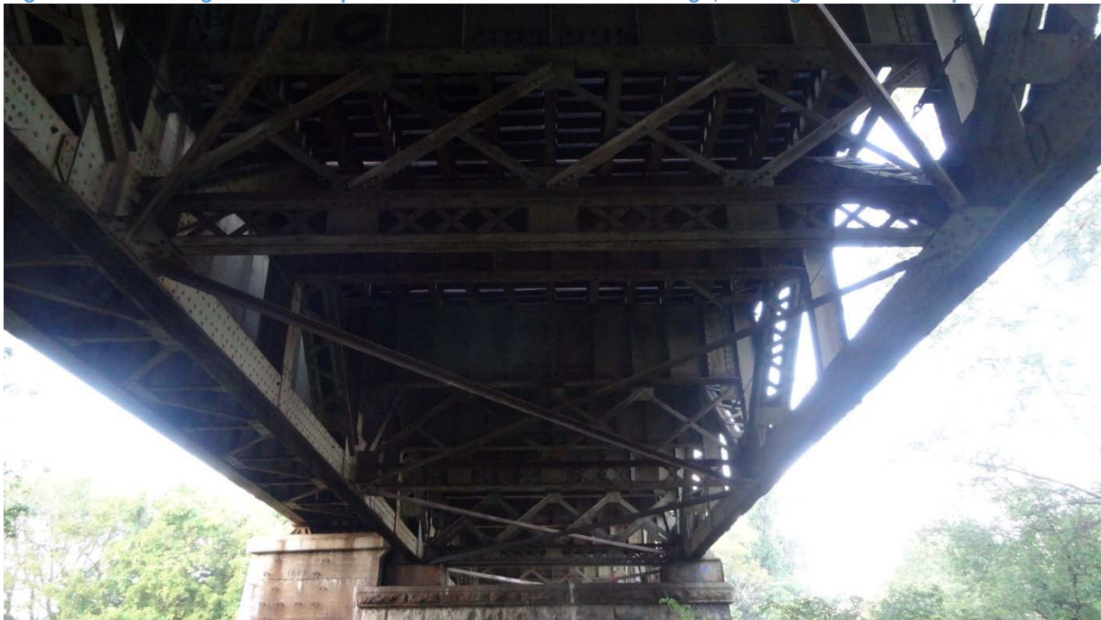
Figure 9-15: Bracing in eastern span of northern Warren truss bridge, looking west towards pier.
