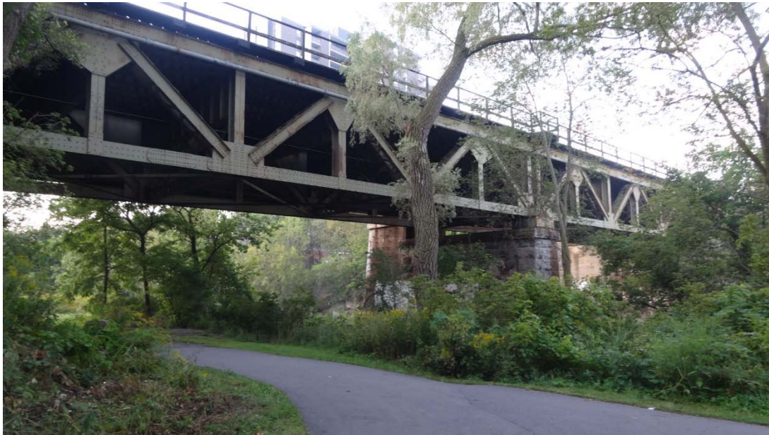
Figure-1-2: North Elevation of the Etobicoke Creek Bridge
