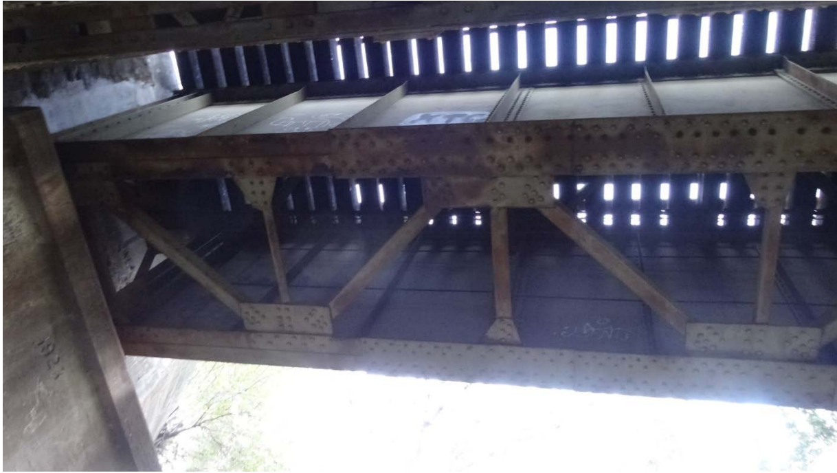
Figure 9-15: Bracing in eastern span of northern Warren truss bridge, looking west towards pier.
