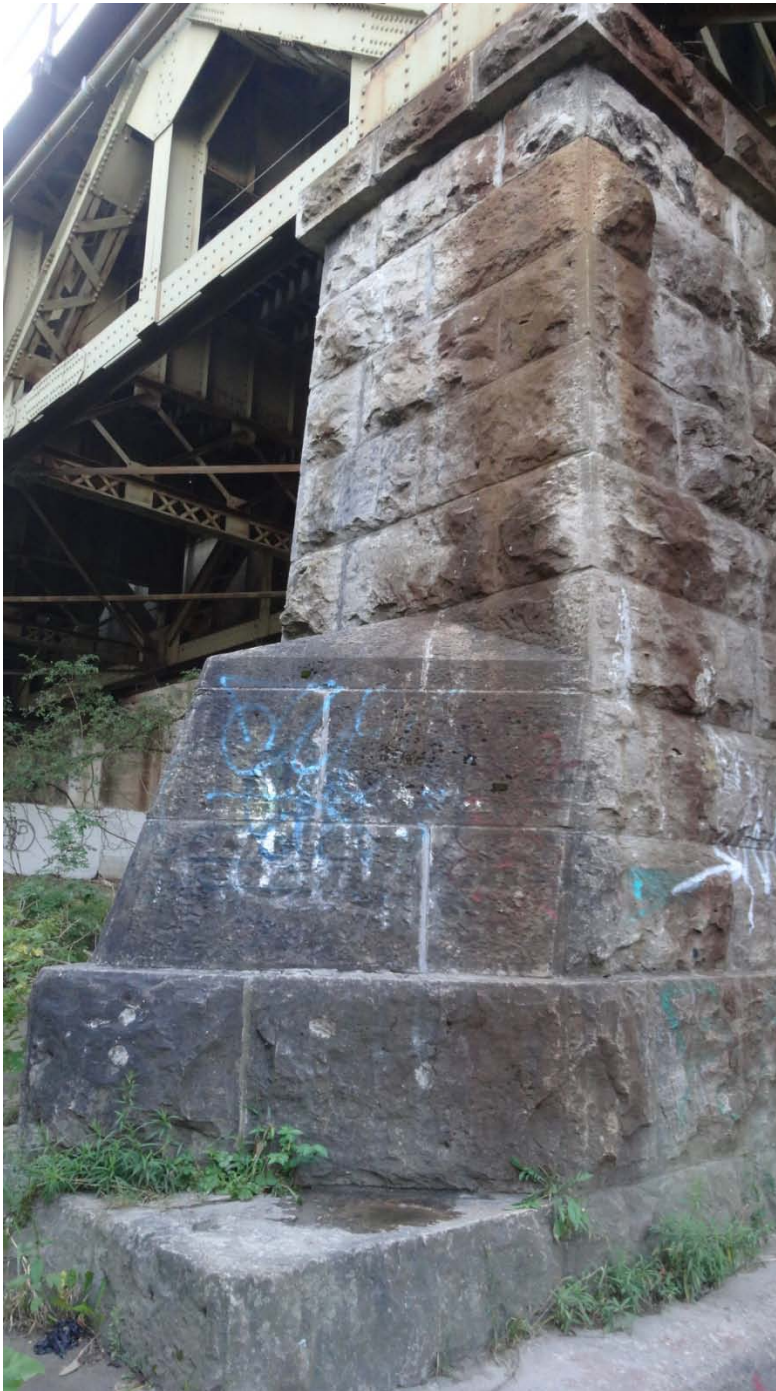
Figure 9-11: North elevation of pier with ice floe protection supporting Warren truss structure, looking southeast.
