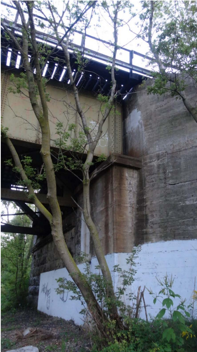
Figure 9-22: East abutment and south elevation of plate girder bridge, looking northeast.
