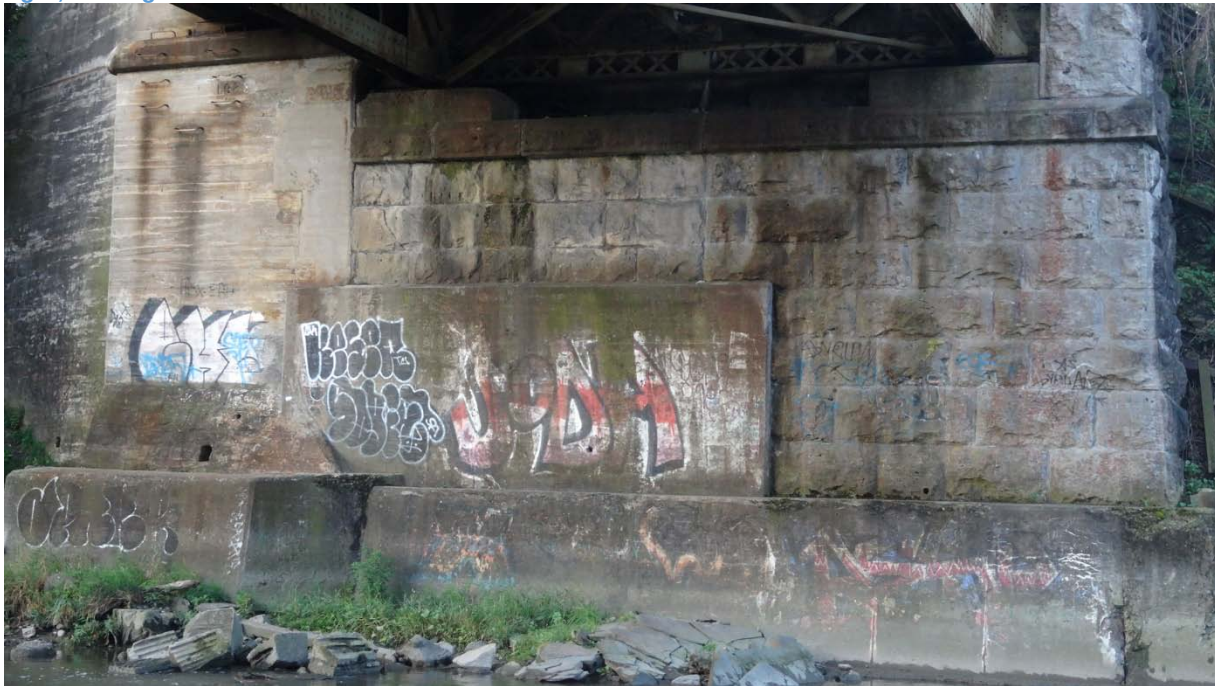
Figure 9-18: West abutment with 1923 plate girder portion at left and 1903 Warren truss at right, looking west.
