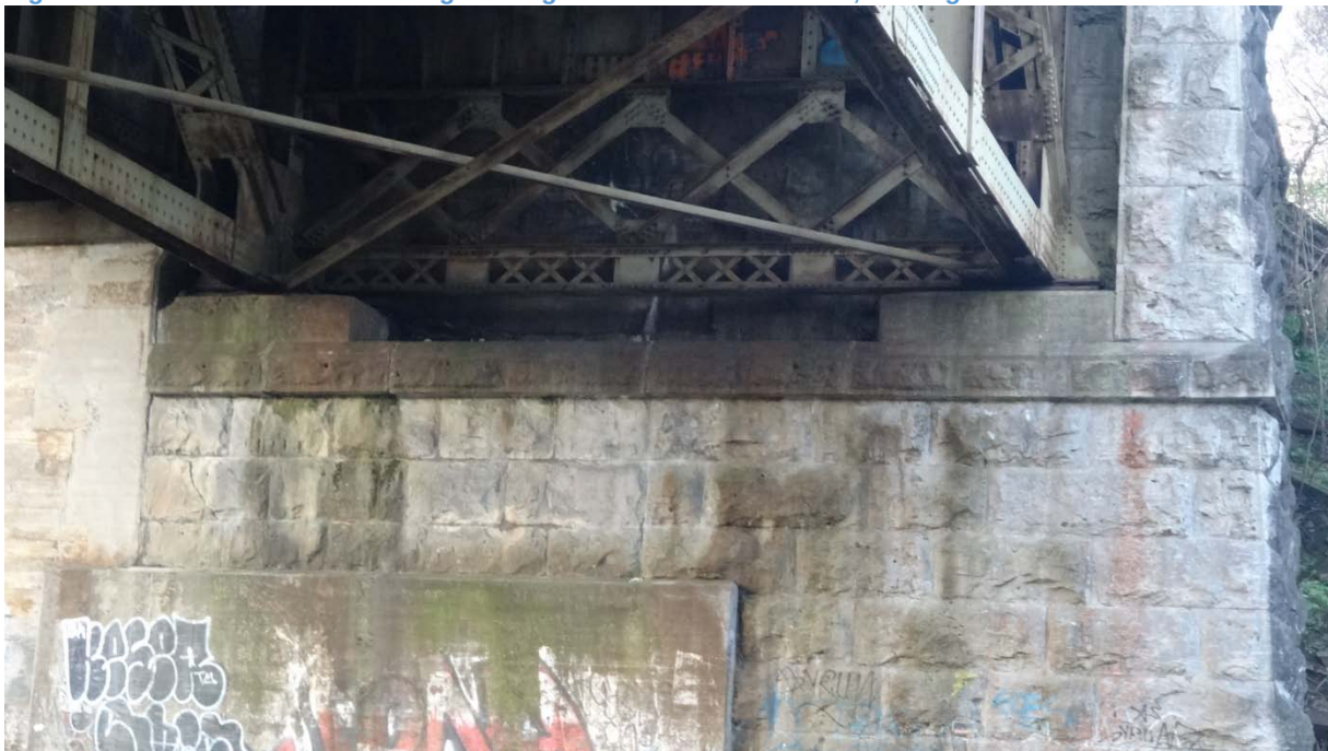
Figure 9-19: East abutment showing bearings on 1903 stone section, looking west.
