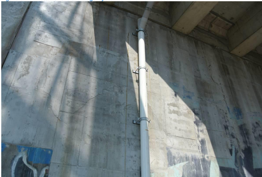
Figure 9-20: Detail of the drainage system on the northwest abutment.
