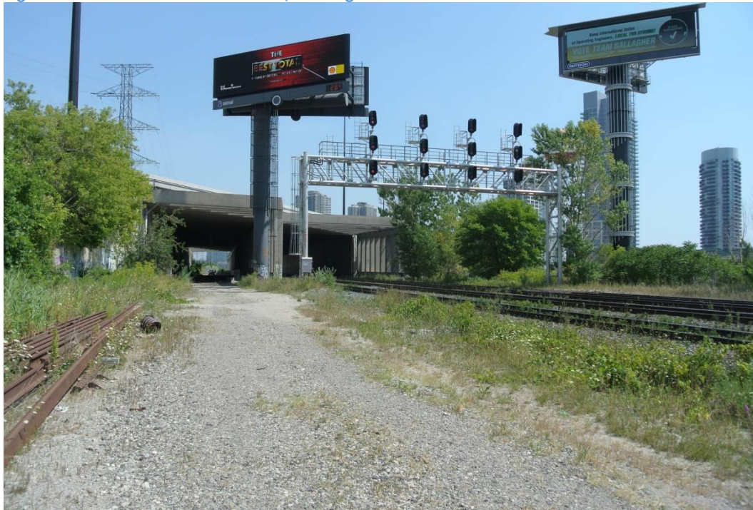
Figure 9-15: View of west elevation, looking east.
