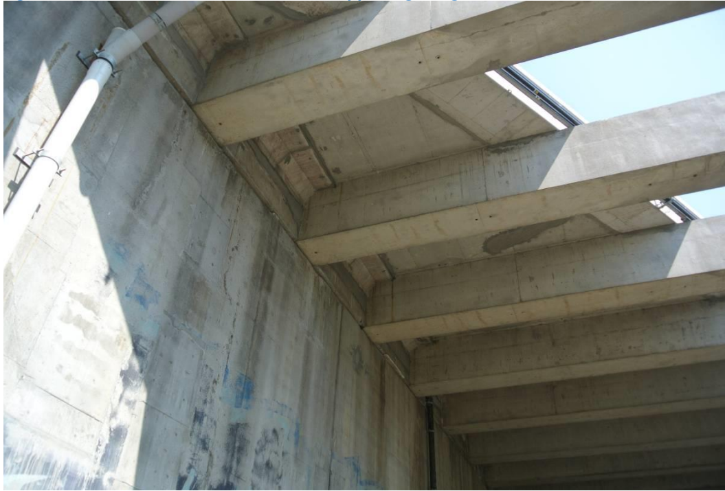
Figure 9-20: Detail of the drainage system on the northwest abutment.
