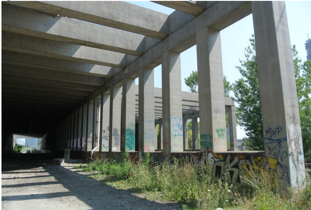
Figure 9-16: View toward west concrete columns, looking east.
