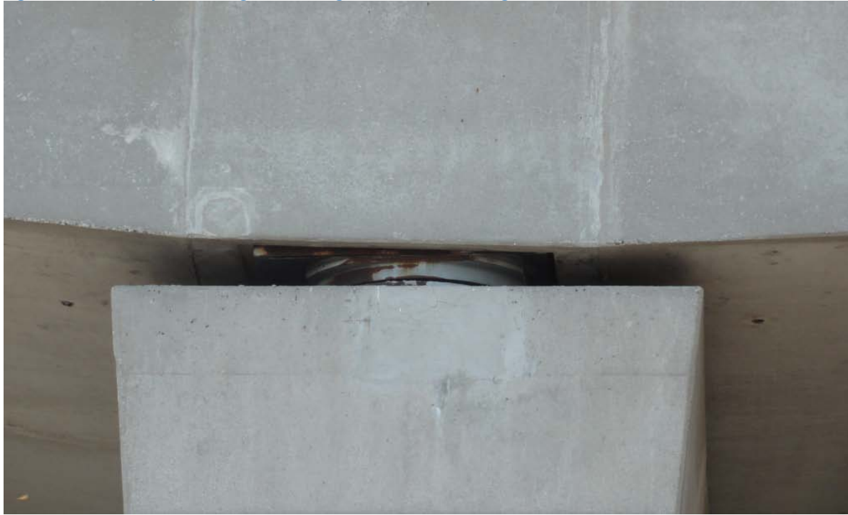
Figure 9-24: Pier B and bridge deck underside showing soot from diesel engines passing underneath, looking south at the Willowbrook Maintenance Facility.
