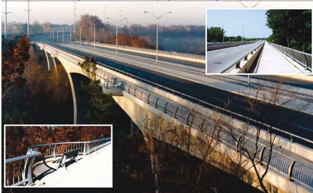
Figure 9-34: Six span precast prestressed concrete Burnhamthorpe Road Bridge over the Credit River, Mississauga, constructed in 1979 (City of Mississauga 2007).
