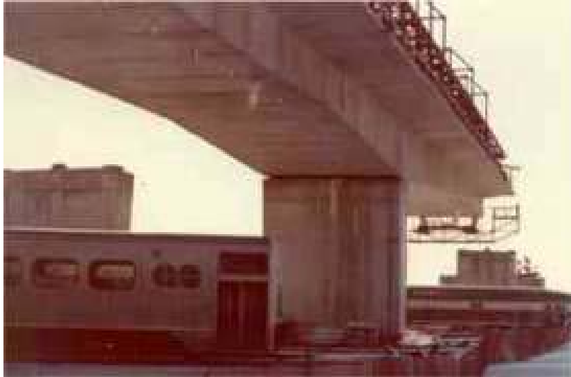
Figure 9-7: Construction of the Islington Avenue Bridge (Planmac Inc.)
