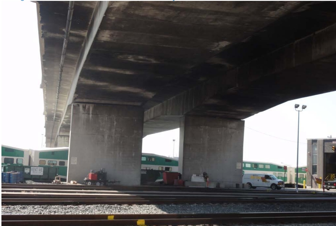
Figure 9-24: Pier B and bridge deck underside showing soot from diesel engines passing underneath, looking south at the Willowbrook Maintenance Facility.
