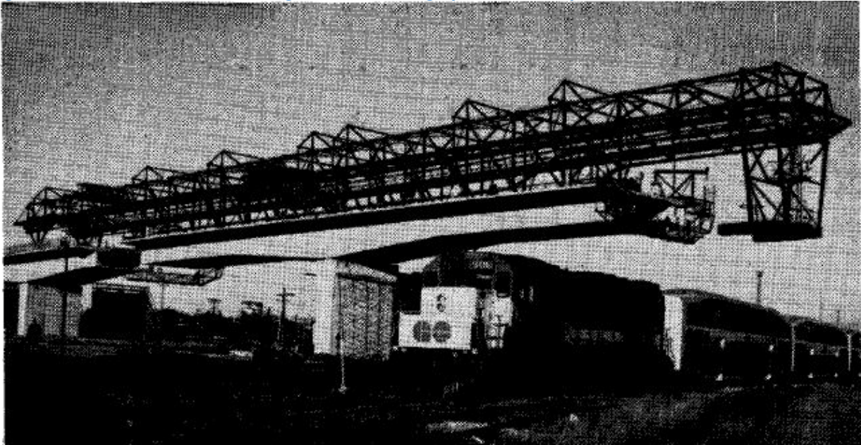
Figure 9-12: Construction of the Islington Avenue Bridge (Lovell 1980:52)
