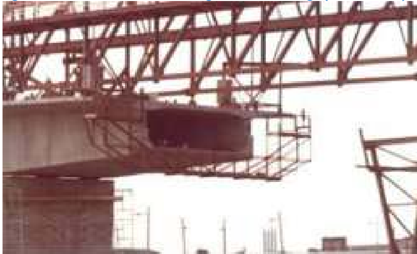
Figure 9-8: Construction of the Islington Avenue Bridge (Planmac Inc.)
