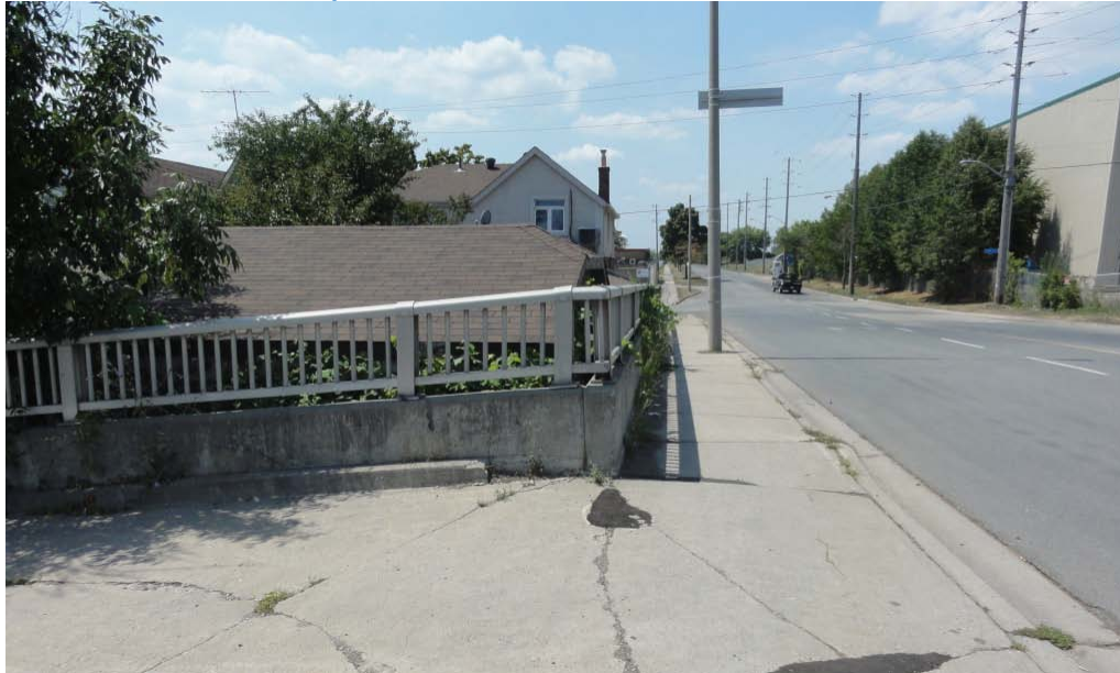
Figure 9-33: Impacts of raising grade level on southern bridge approach, looking west down New Toronto Street from Islington Avenue. Note the tall retaining wall at left and the roof level of the residence compared to street level.
