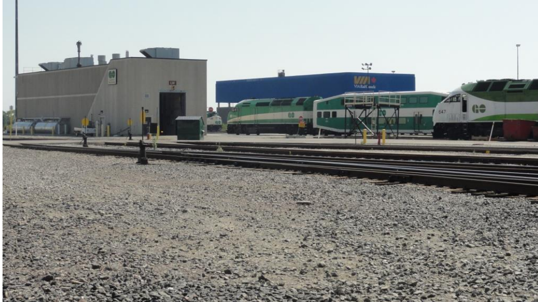
Figure 9-12: Study area showing Locomotive Wash (LW) building, tracks, and trains, looking southeast. Note the Via Rail maintenance facility at rear center.
