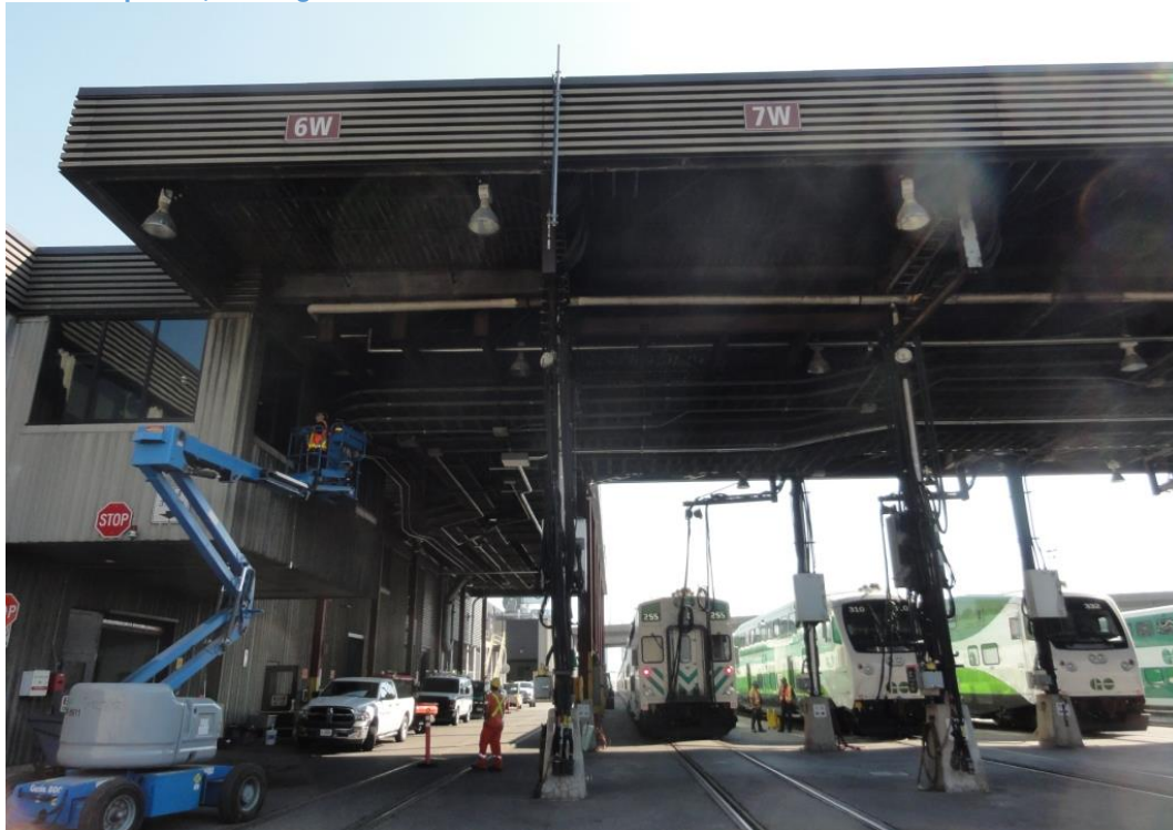
Figure 9-21: Auxiliary power canopy in southern yard, with trains hooked to auxiliary electrical power, looking northeast.
