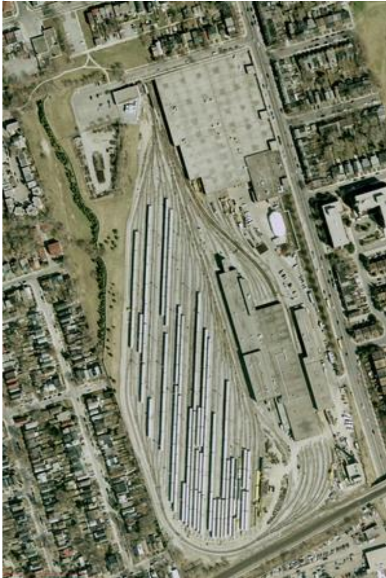
Figure 9-38: TTC's Greenwood Subway Yard from satellite imagery. (Transit Adel and Bow 2015)
