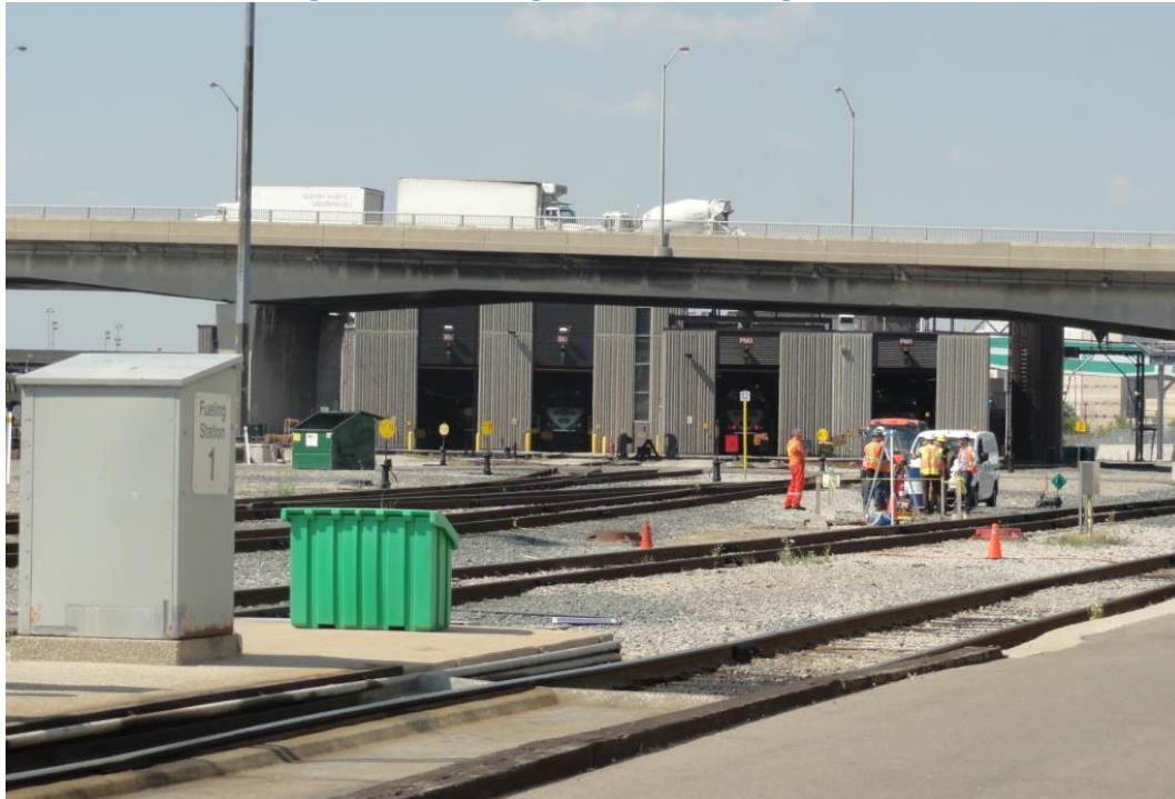
Figure 9-21: Auxiliary power canopy in southern yard, with trains hooked to auxiliary electrical power, looking northeast.
