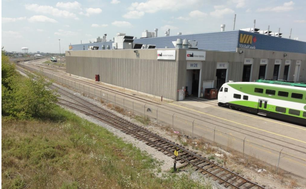
Figure 9-36: Via Rail Toronto Maintenance Facility, looking southwest from the Islington Avenue Bridge.
