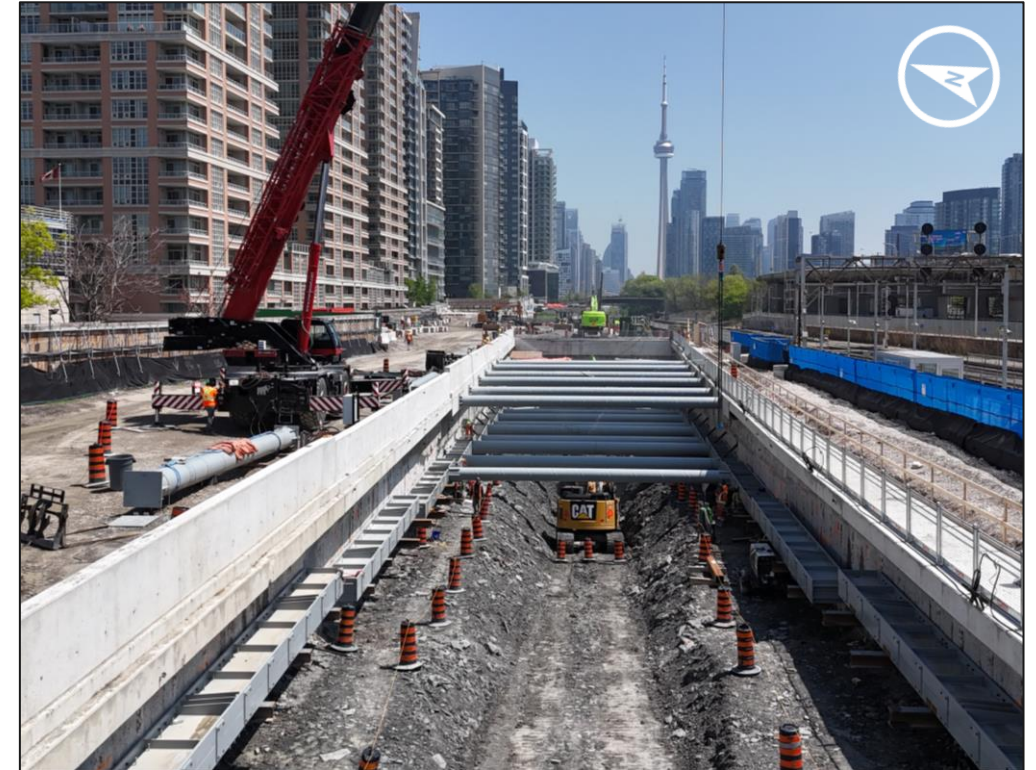
Ontario Line portal walls and steel struts, ensuring structural integrity as crews excavate.
