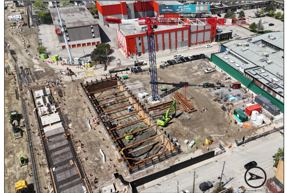
Structural support beams being installed to support the future north main entrance building.
