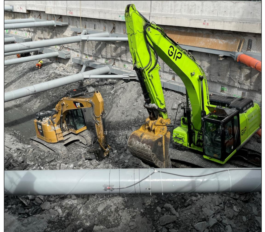
Ontario Line portal being excavated.
