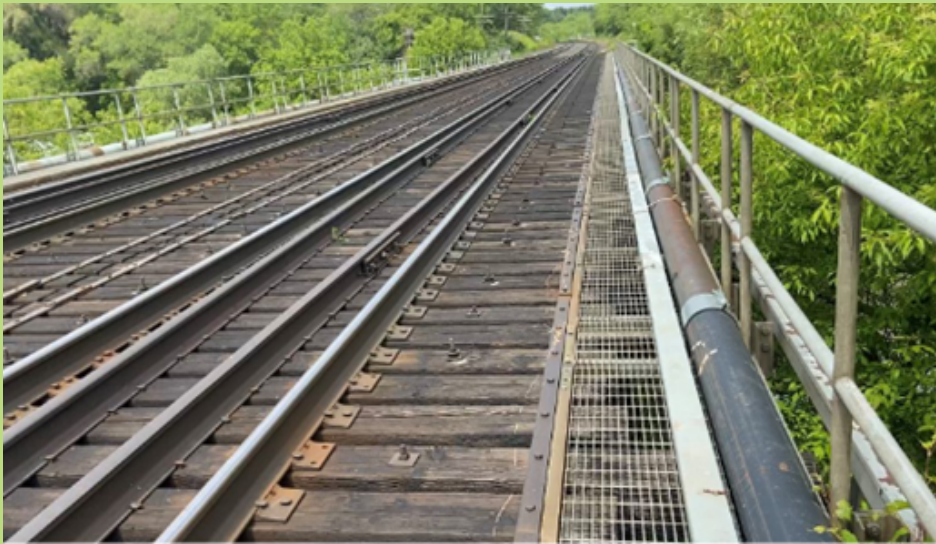
The bridge's timber deck ties and track will be replaced. (Metrolinx image).
