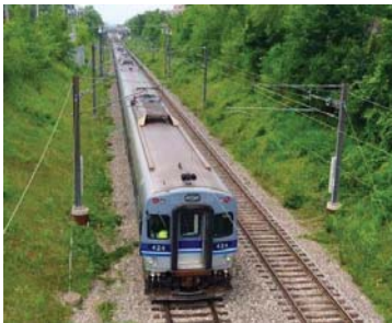
Location: Montreal AMT - Deux-Montagnes line
