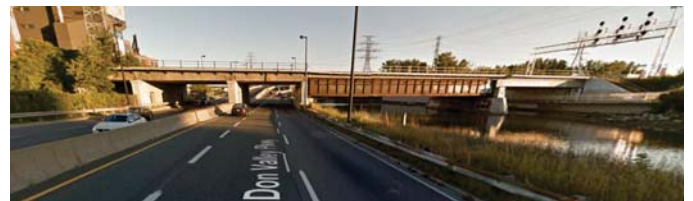
Don Valley Parkway and Don River Bridges (looking south)
