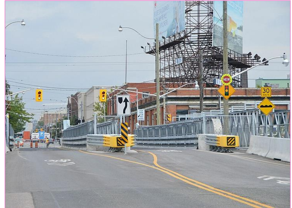
Bridges over the GO Transit Lakeshore West Line, on Dufferin Street.
