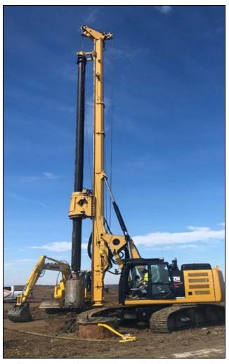
**Drilling rigs** bore deep holes into the ground for foundational supports.
