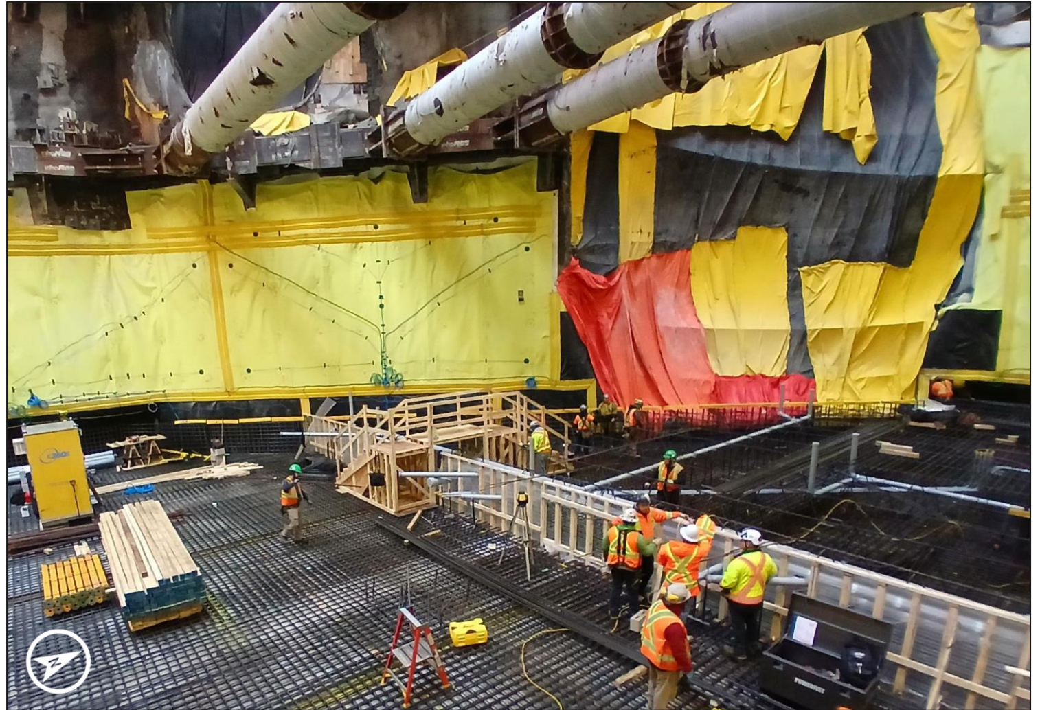
View of the rebar installation from the south site
