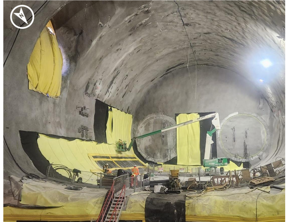
Cavern view facing the south headwall
