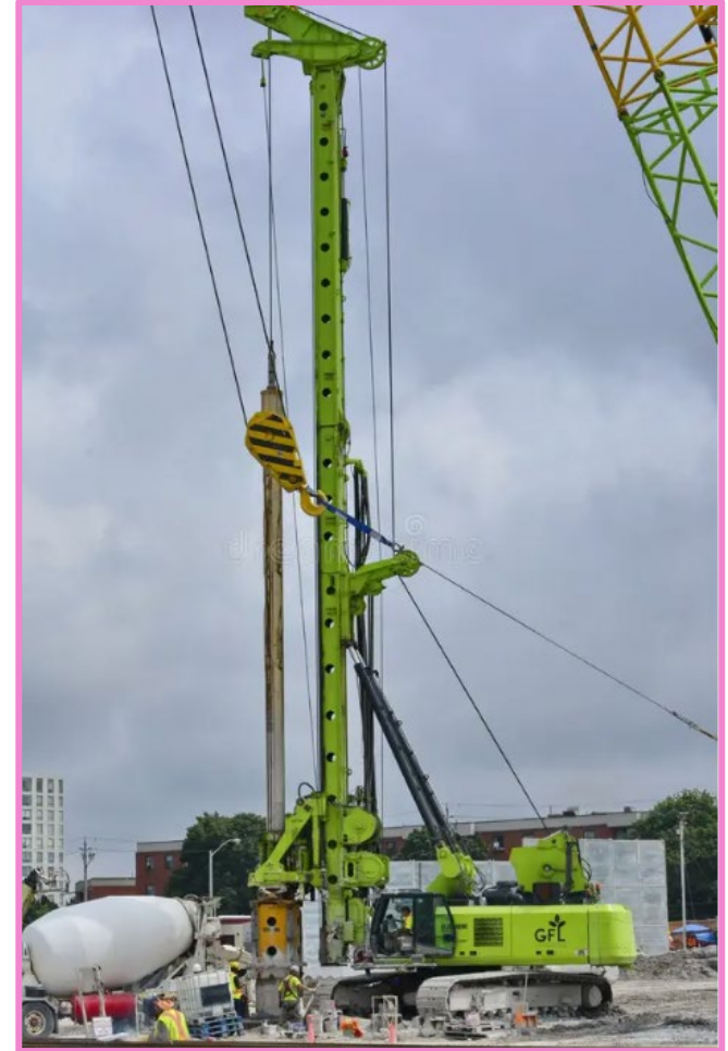
Drilling machine used in pile construction.
