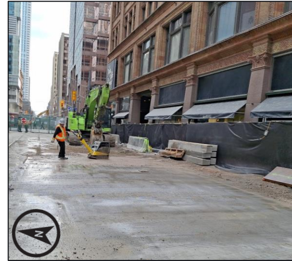
Piling platform at the Queen west station site
