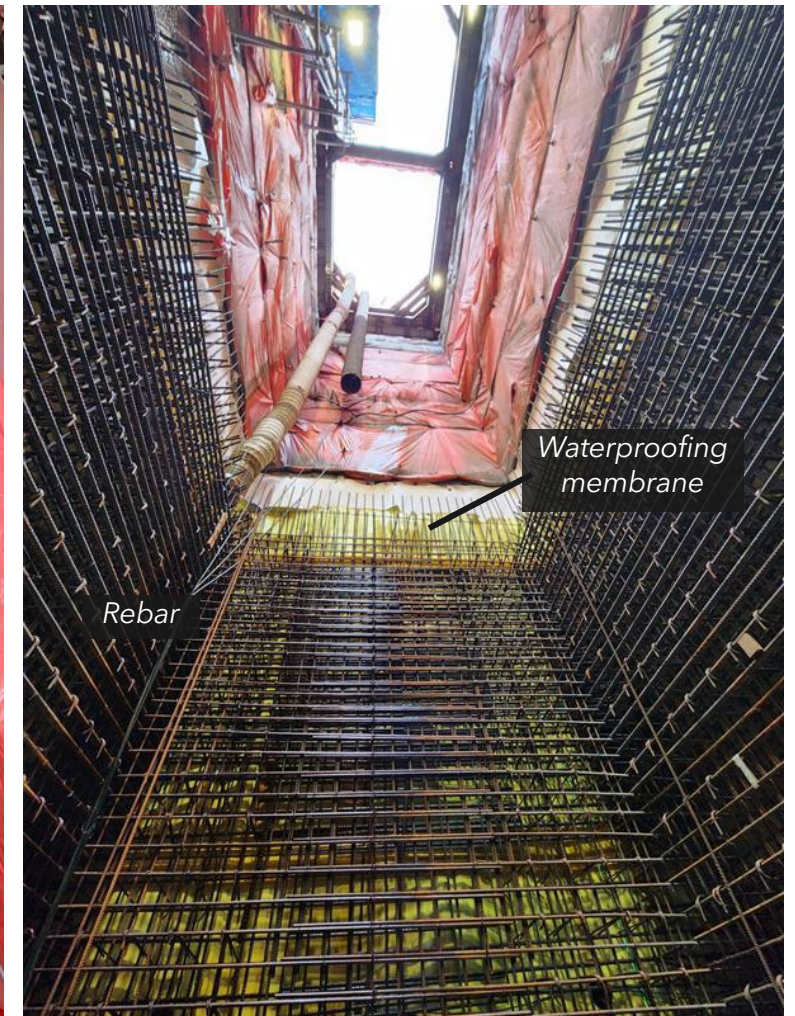
Looking up the shaft at the rebar installation.
