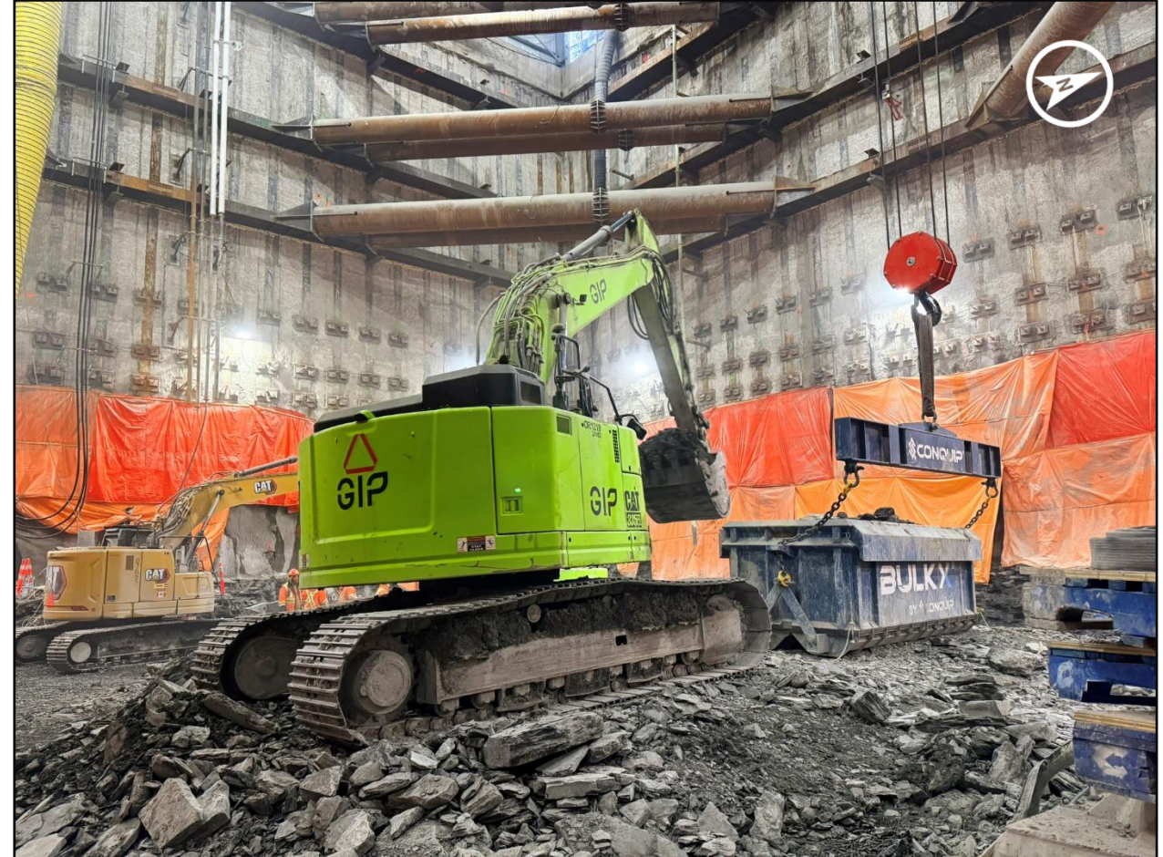
Excavator loading shale into the skip bin
