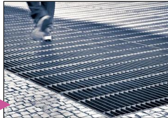
Example of a vent shaft. Visible metal grates integrated into the sidewalk.
