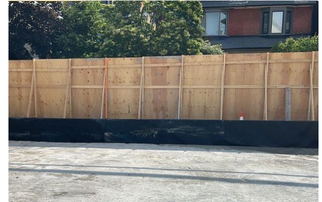
Raised curb and Geotextile Fabric:
