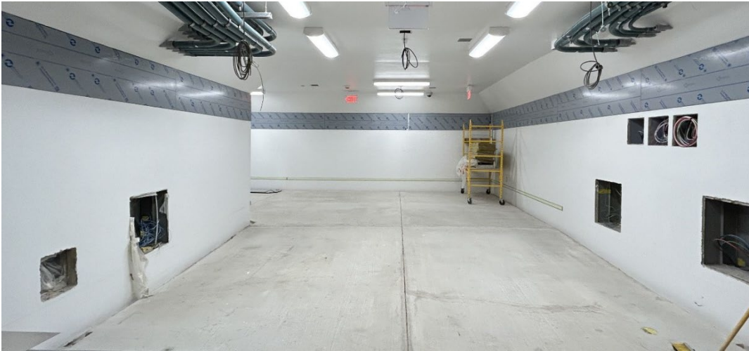
Figure 2: New pedestrian pavilion/tunnel at the end of Randolph Ave
