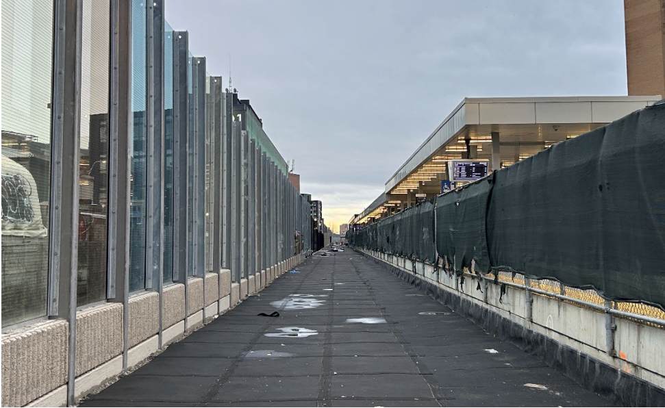
Figure 3: Railpath Ernest Avenue facing Dundas St
