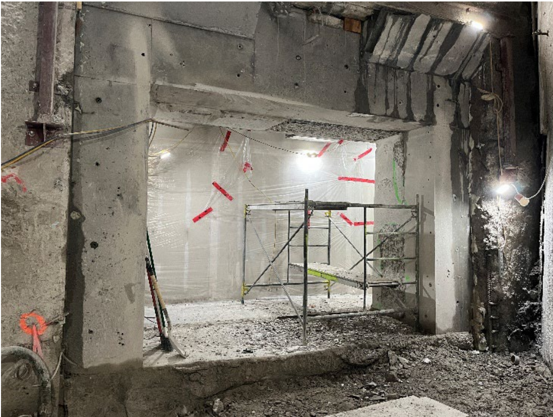
Figure 1: Westbound Platform Opening
