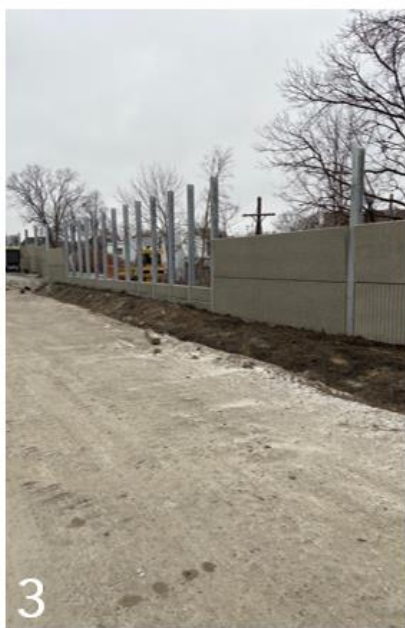
3 & 4. Noise Barrier Wall Construction
