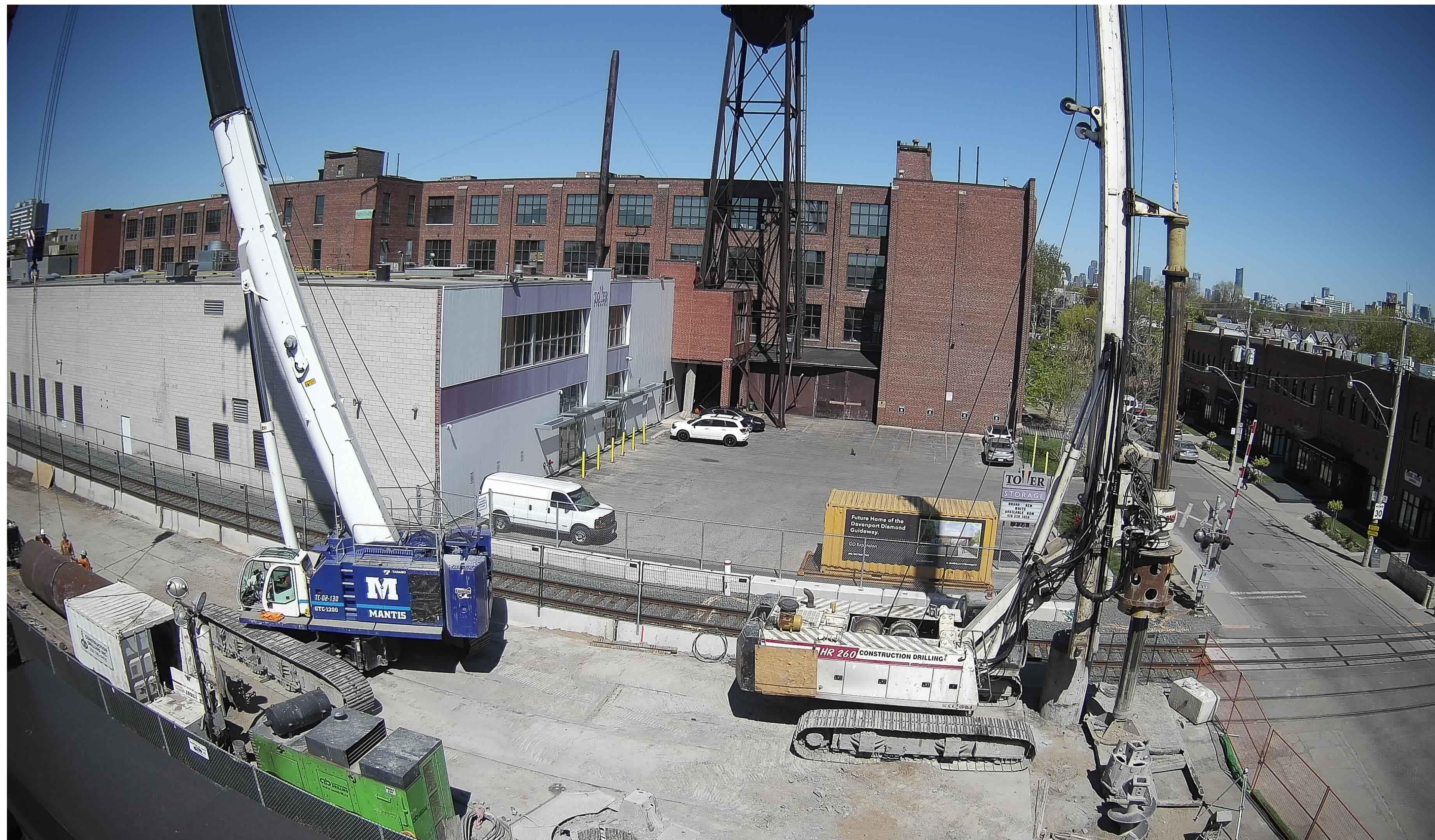
Caisson drilling at Wallace Ave.
