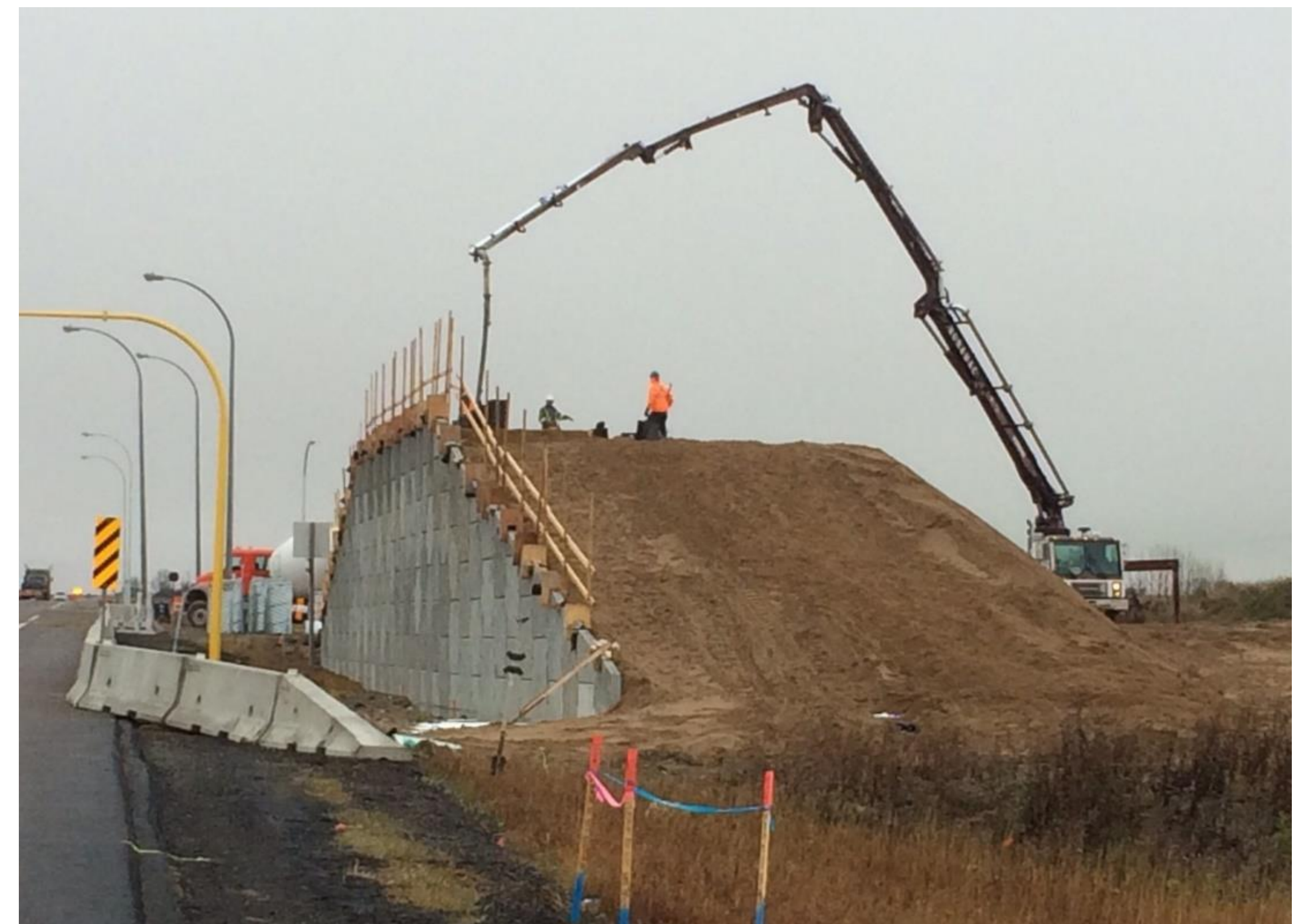
A closer look at an MSE wall (photo credit: Regina Bypass).
