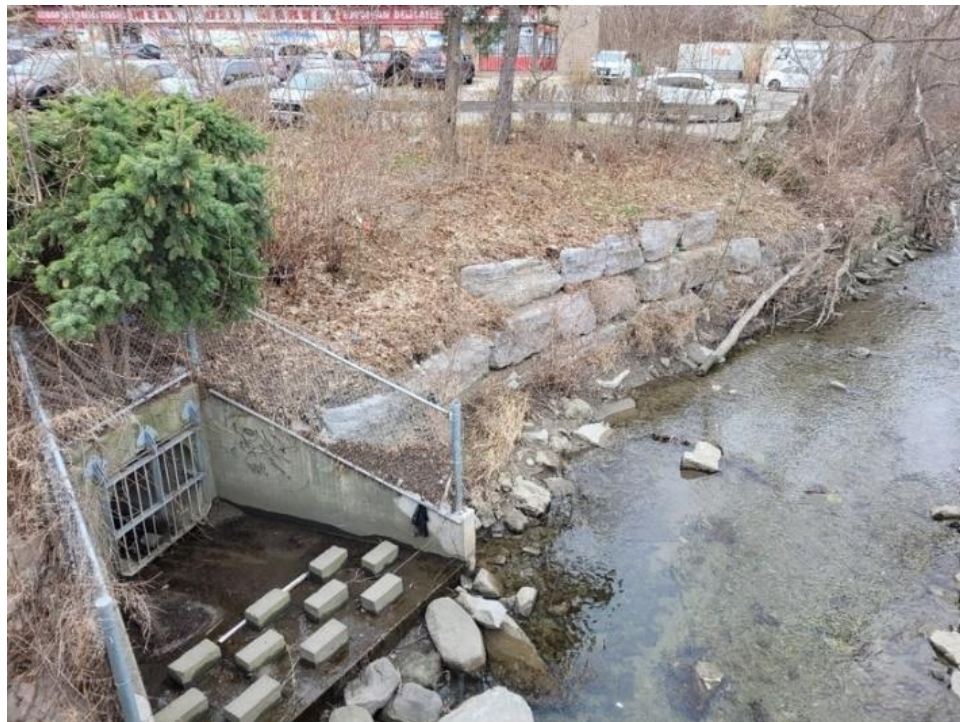
Photo 12: Conditions around Little Etobicoke Creek, banks heavily sloped and reinforced to prevent erosion, facing north (March 31, 2021)
