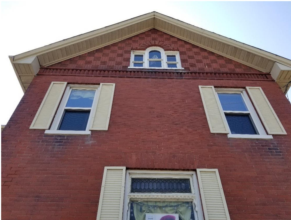
Plate 7: View of basketweave brickwork beneath the gable end on the northern elevation (ASI 2021).
