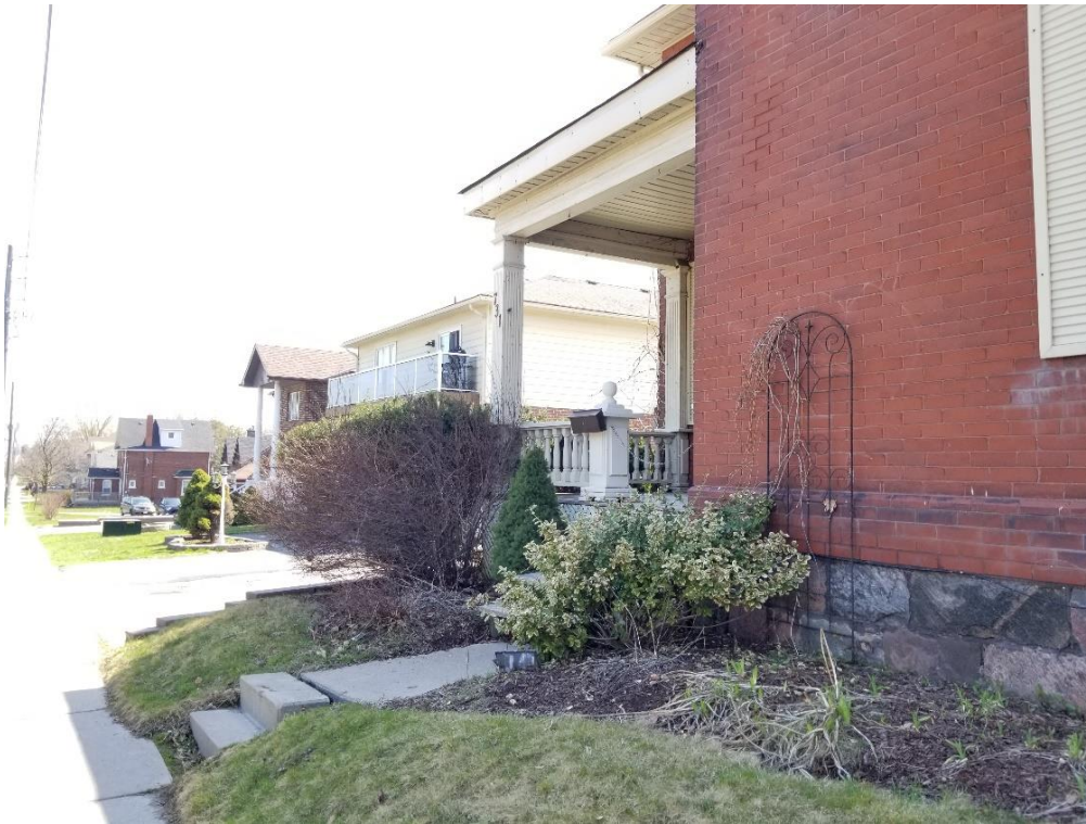
Plate 9: View of the front porch and fieldstone foundation (ASI 2021).
