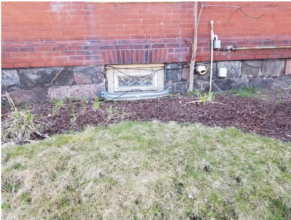
Plate 10: View of the basement window, wash course, and fieldstone foundation (ASI 2021).
