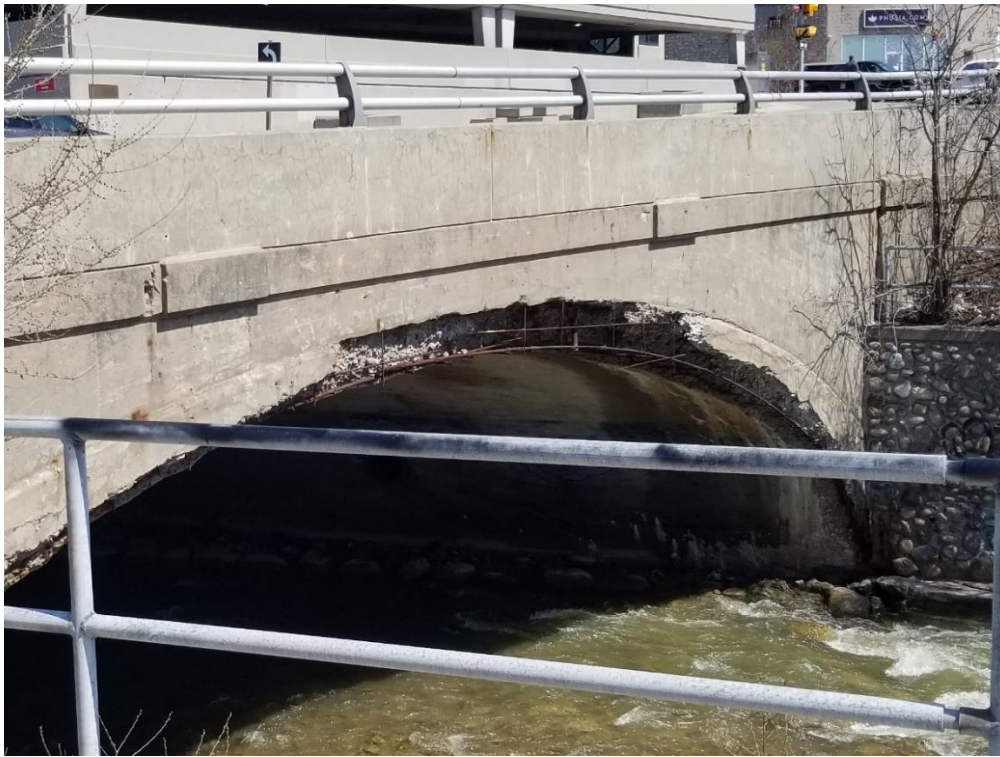
Plate 7: View of the spalling and exposed rebar on the southern elevation (ASI 2021).
