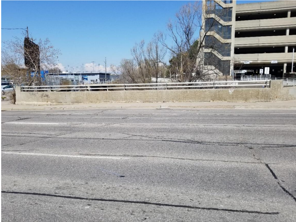
Plate 6: Northern barrier system and parapet wall (ASI 2021).
