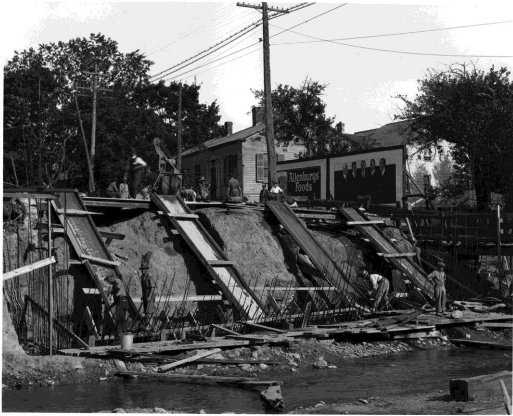
Figure 17: Photograph of the construction of the King Street West Bridge (Anonymous, 1921)
