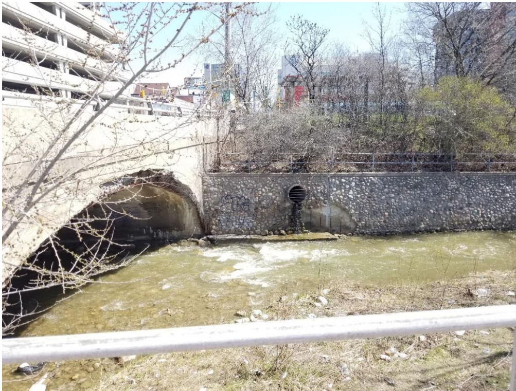
Plate 3: Southeast abutment and retaining wall (ASI 2021).
