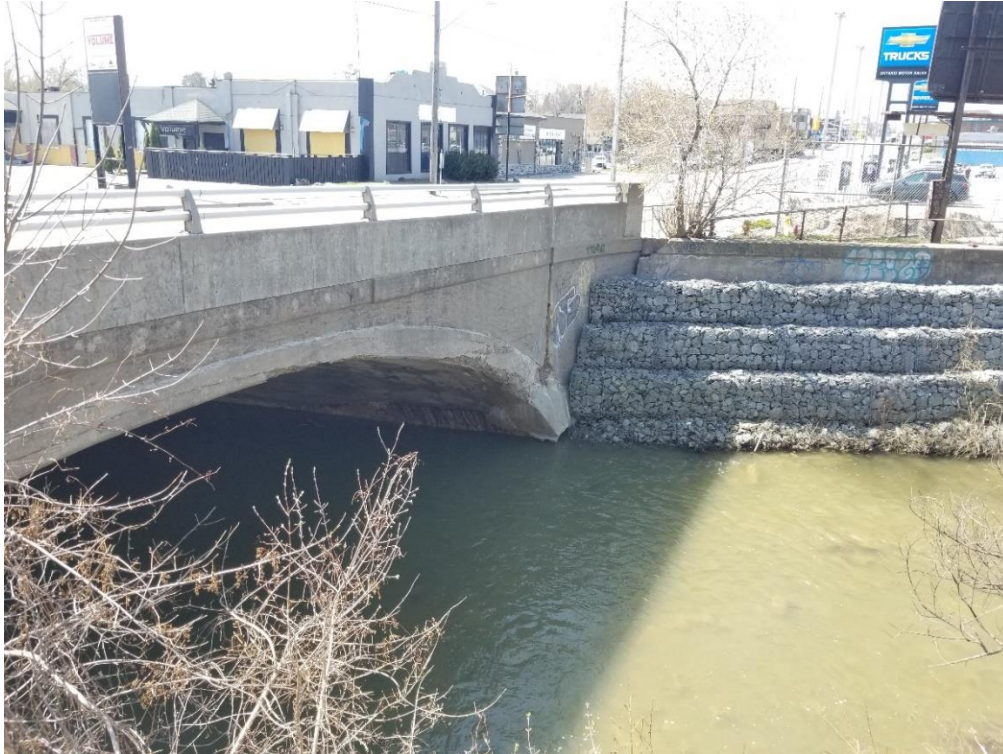
Plate 4: Northwest abutment and retaining wall with gabion baskets (ASI 2021).
