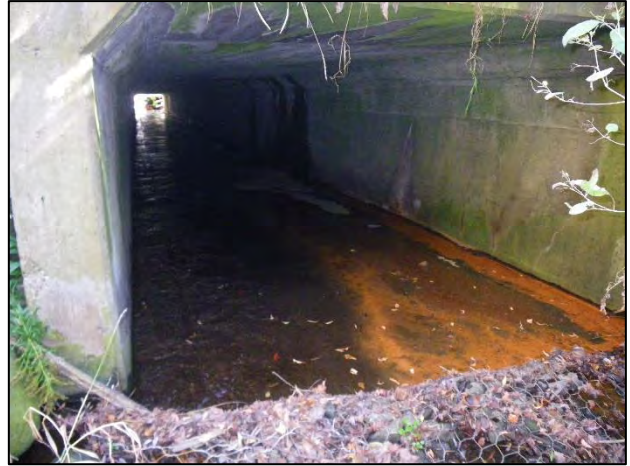
Crossing 10: Facing south (downstream) at the Kingston Road culvert. Note gabion basket in foreground and water level drop to concrete floor, then sheet flow.
