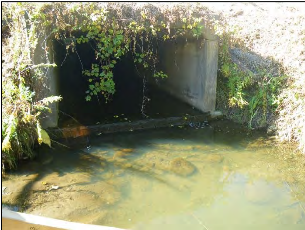
Crossing 10: Facing north (upstream) at the downstream end of the Kingston Road culvert. Note pool with Creek Chub and drop at lip of culvert.
