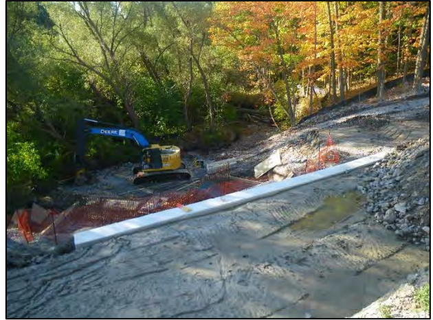
Crossing 2: Facing south (downstream) at downstream end of Ellesmere Road culvert and active construction area where it is being extended.
