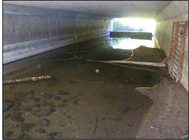
Crossing 19: Facing north (upstream) inside west cell of culvert. Note baffles and trapped sediments.
