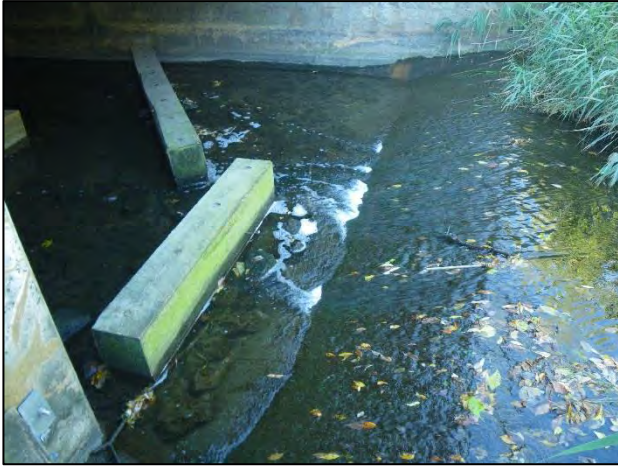
Crossing 19: Facing west at the concrete drop into the west cell of the culvert. Note baffles..
