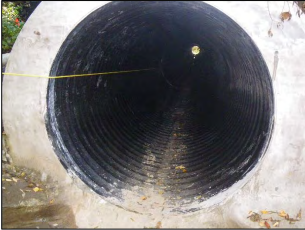
Crossing 2: Facing south (downstream) at upstream end of Ellesmere Road culvert. Note lack of flow and new lining.
