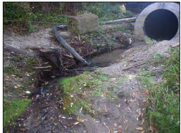
Crossing 2: Facing south (downstream) at upstream end of Ellesmere Road culvert. Note flow bypass and new culvert lining.
