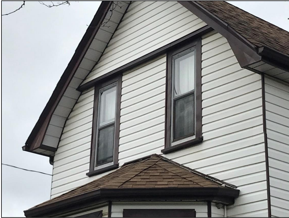
Plate 4: Detail of vinyl cladding and window surrounds on gable end of 3344 Ellesmere Road (ASI 2021).
