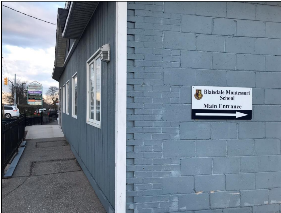
Plate 3: Detail of northwest corner showing concrete masonry units and brick likely indicating a brick façade beneath the wood siding on the north elevation (ASI 2021).
