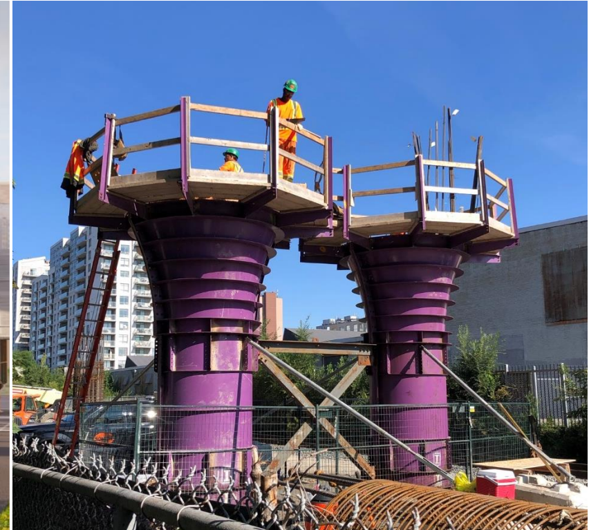
Bridge pier formwork on the site
