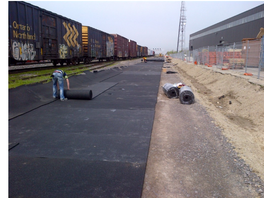
Example of ballast mat installation
