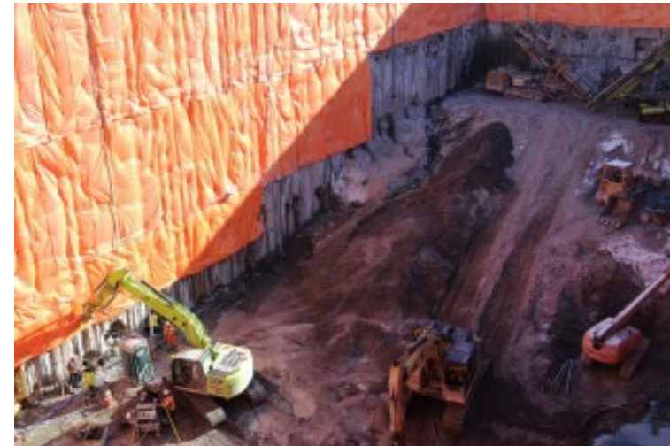
Example of Excavation Support. Source: Metrolinx
