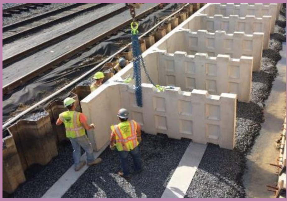
T-wall construction example
