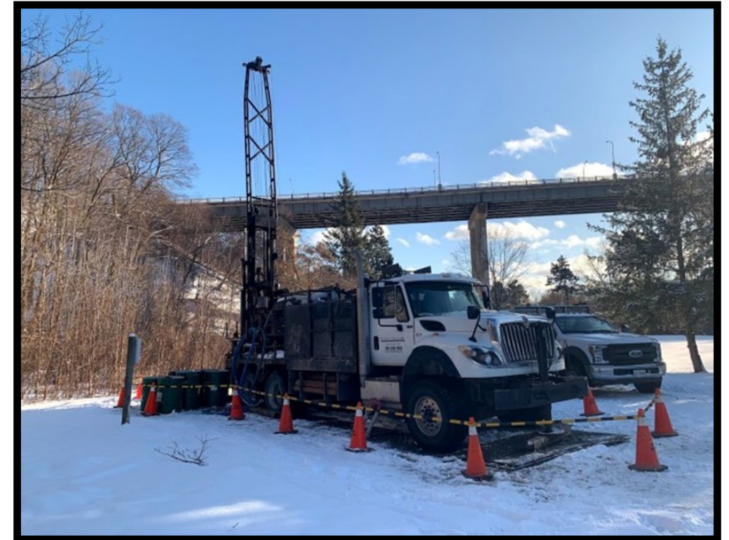
Core sample and truck-mounted drill rig
