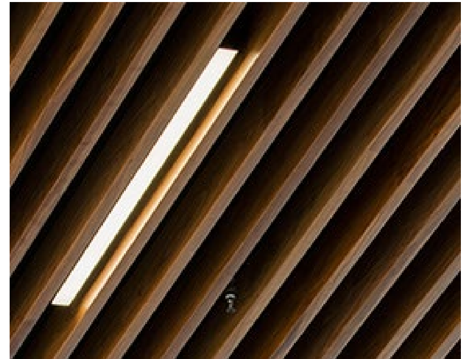
Wood baffles ceiling
