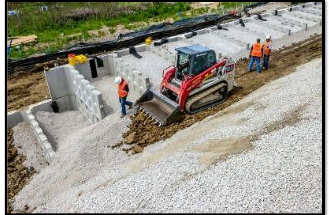
Example of T-wall construction
