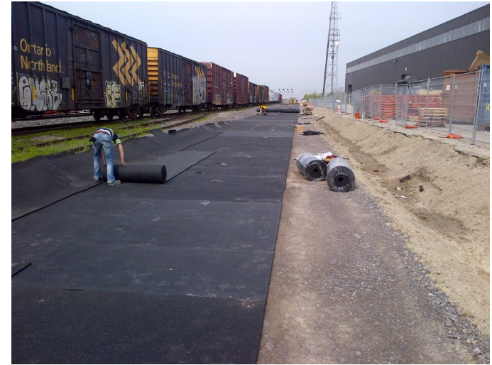
Example of ballast mat installation
