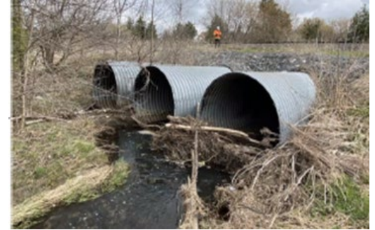
Existing triple-cell CSP culvert
