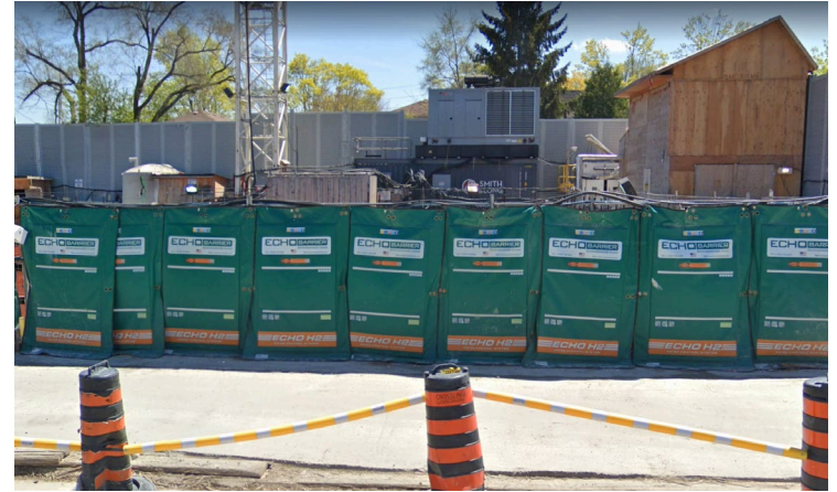
Example of moveable construction noise-absorbing barrier.
