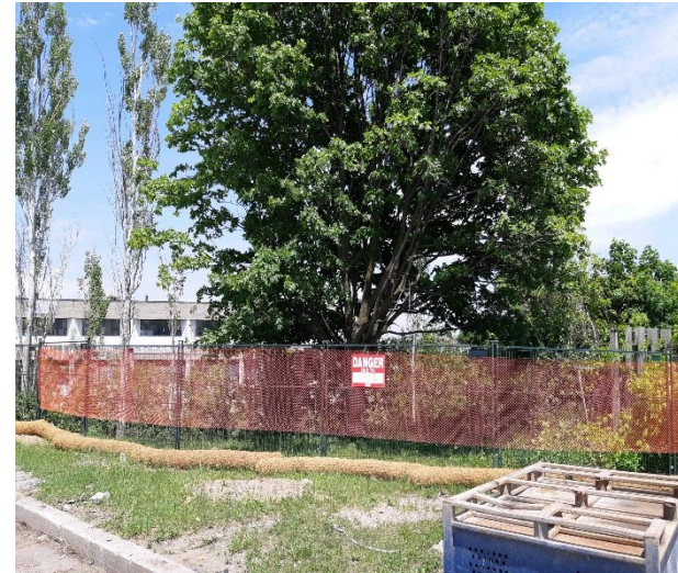
Tree protection fence example
