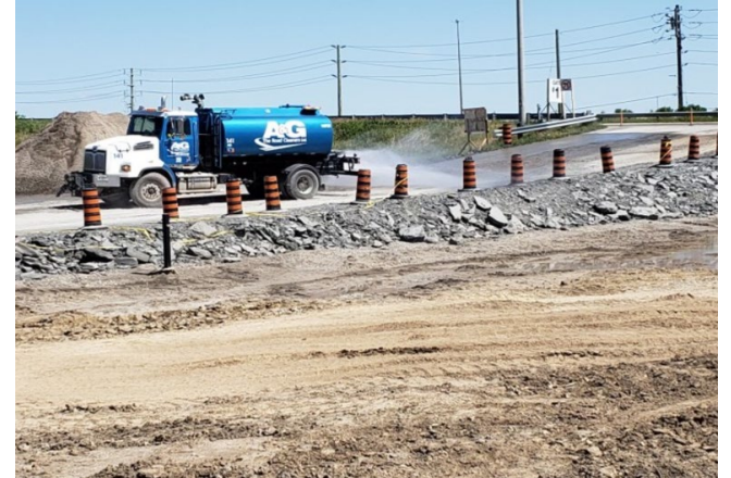
Example of watering truck used for dust suppression
