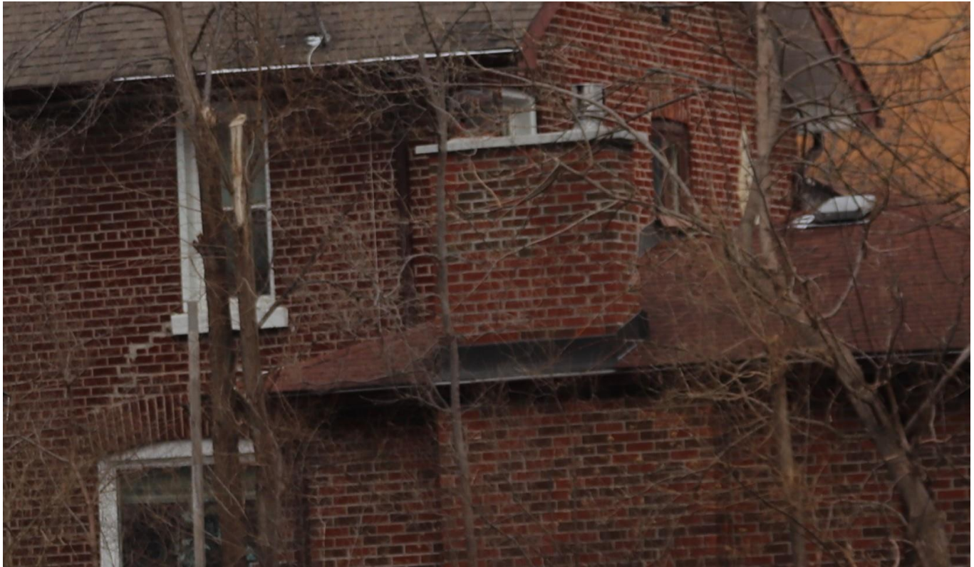
Photograph 9: View of the west elevation, illustrating the red brick chimney containing a concrete crown and metal caps, looking east (AECOM 2021)
