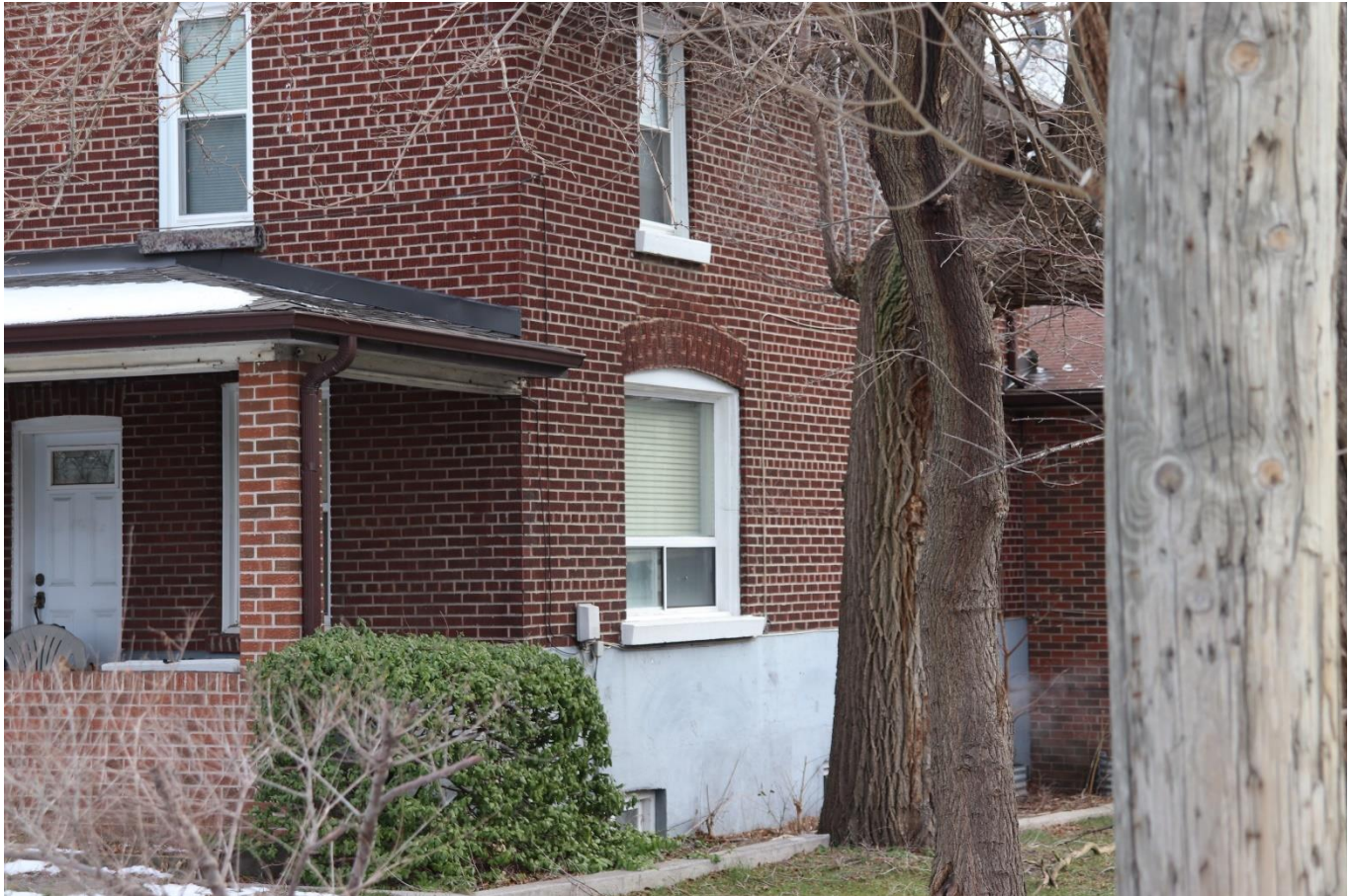
Photograph 8: View of the west elevation, illustrating one of the vinyl bottom sliding windows with a fixed top and brick voussoirs and concrete sills, looking southeast (AECOM 2021)
