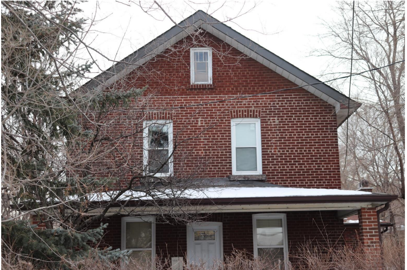
Photograph 4: View of the north elevation, illustrating the two vinyl one-over-one sash windows and the small wooden frame window, looking south (AECOM 2021)
