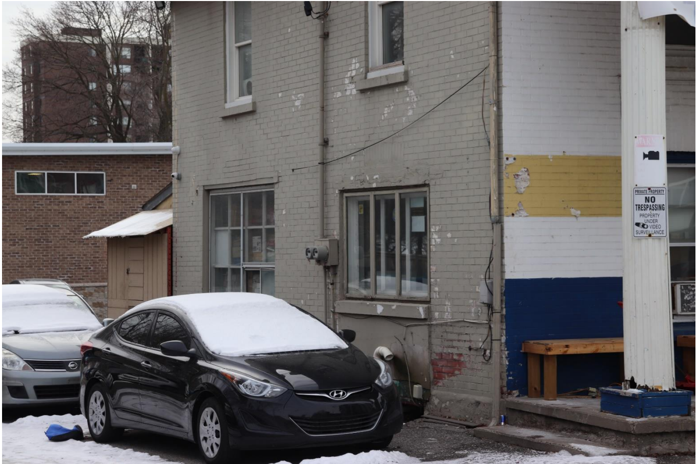
Photograph 11: View of the east elevation illustrating the aluminum three paned sliding window and the twelve-paned aluminum window, looking south (AECOM 2021)
