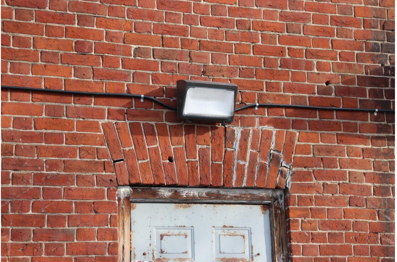
Photograph 4: Detail of jack-arched brick voussoirs above the door opening on west elevation (AECOM, 2021)
