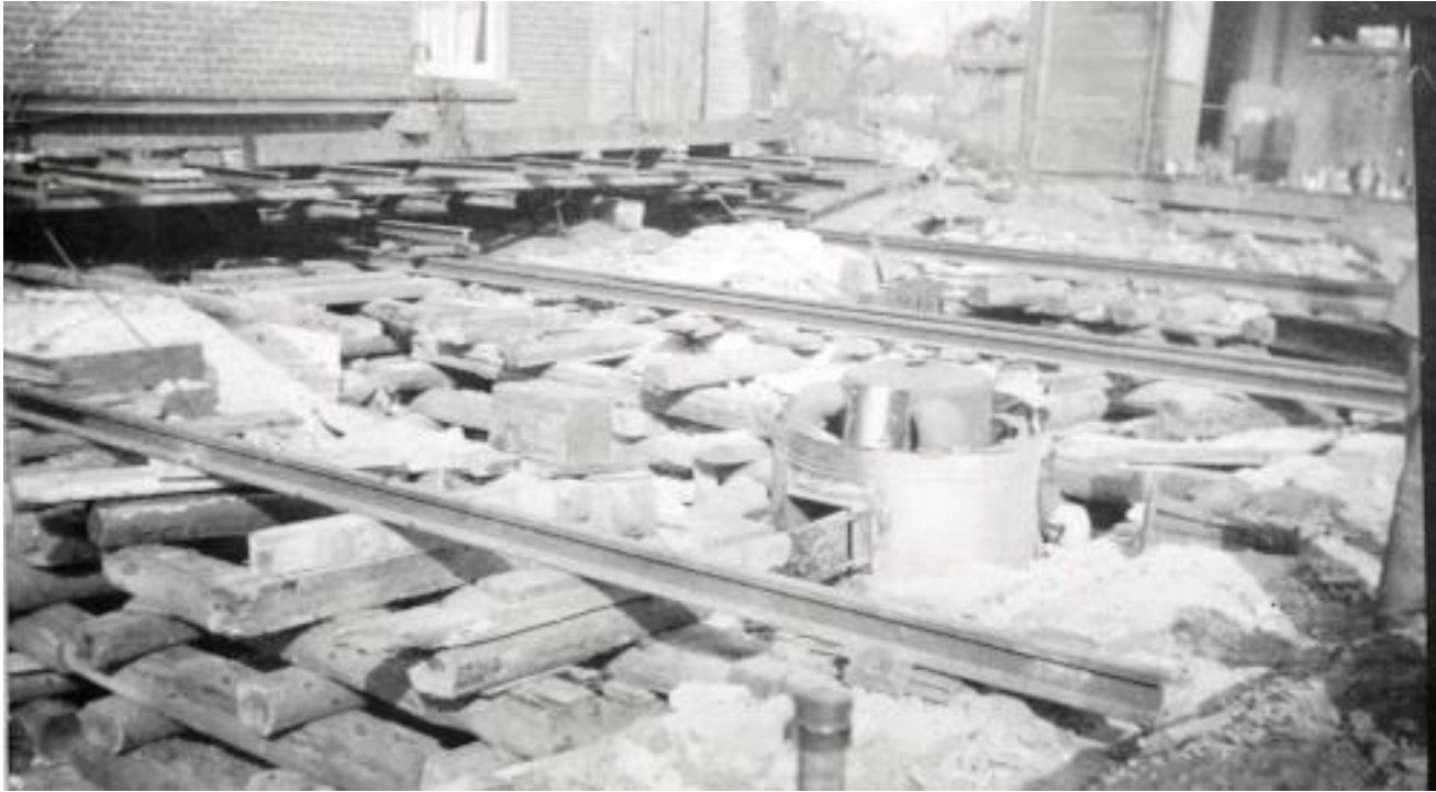
Image 6: Steel rails used to move the building to its new location (Heritage Mississauga)
