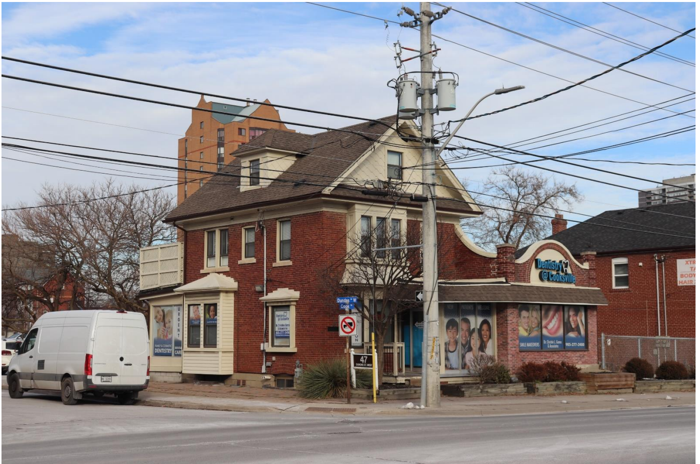
Photograph 3: View of the façade and west elevation of 47 Dundas Street West at the corner of Dundas Street West and Cook Street (AECOM, 2021)
