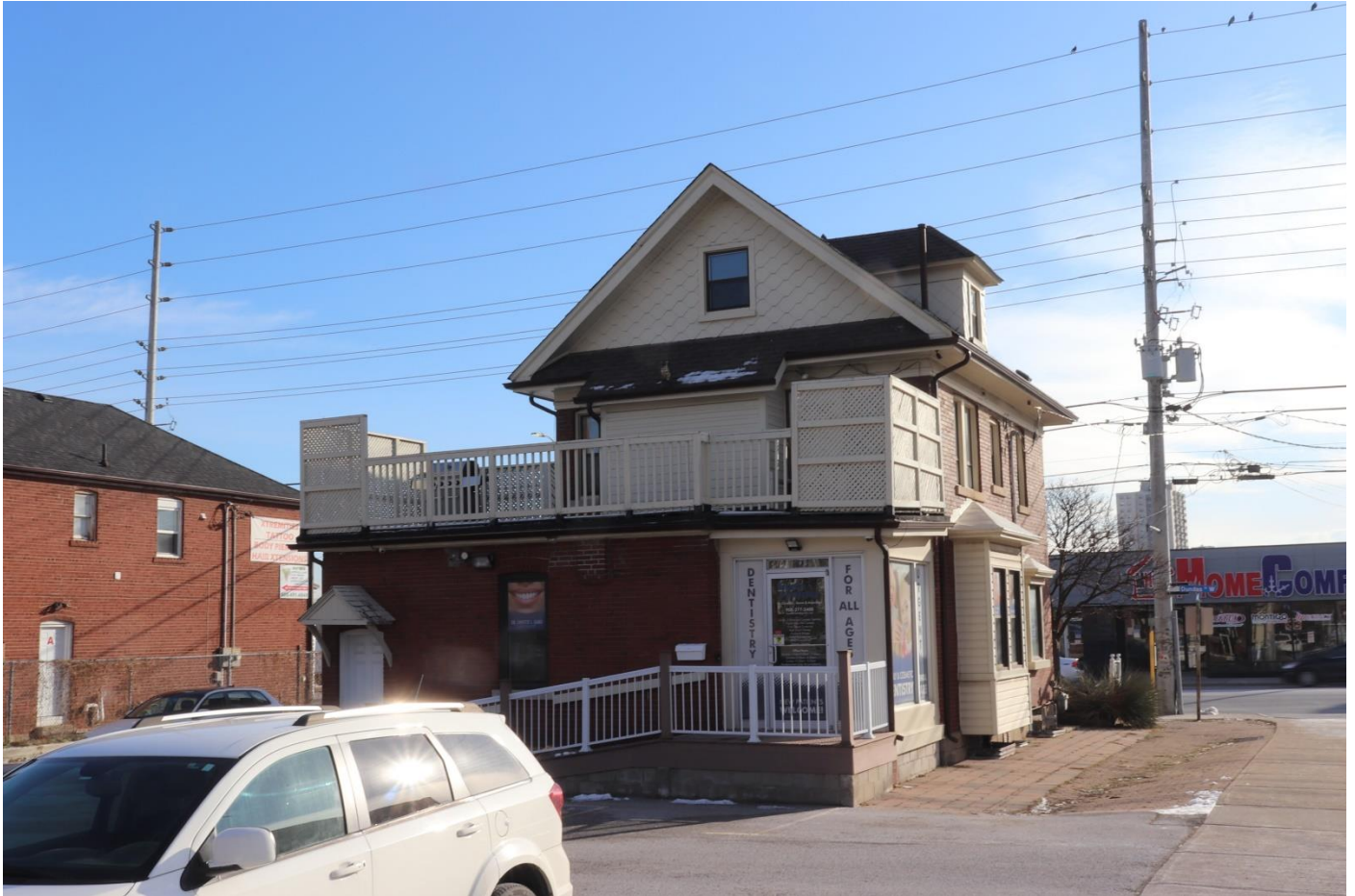
Photograph 6: View of the north elevation (rear) of 47 Dundas Street West (AECOM, 2021)
