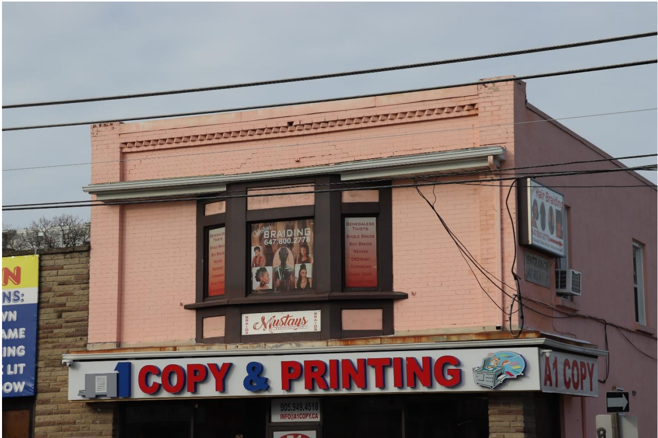
Photograph 2: Close-up view of the second storey of the front façade of 51 Dundas Street West, showing decorative mouse-tooth style brick cornice and pilasters (AECOM, 2021)
