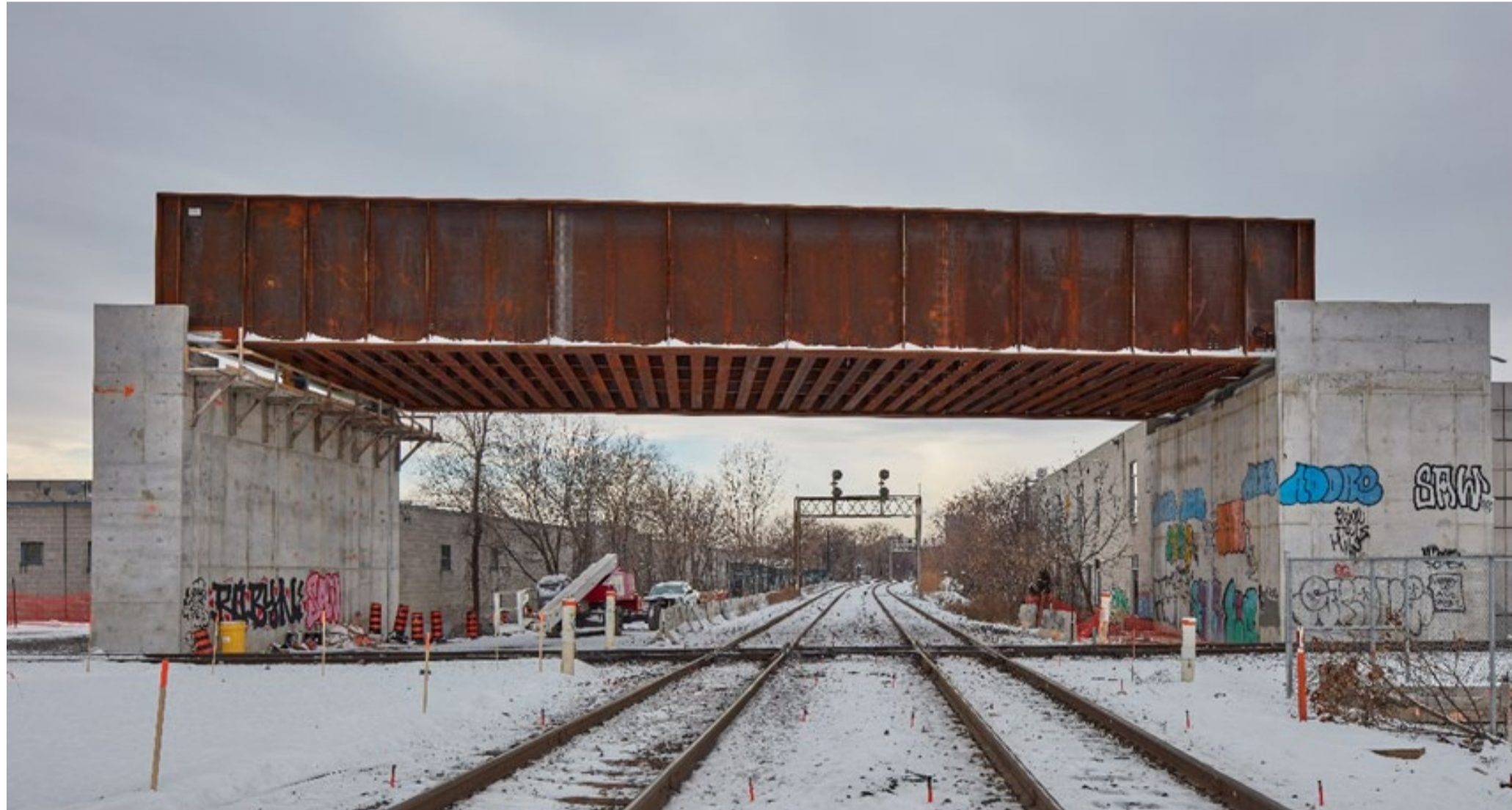
CP bridge girders (looking west).
