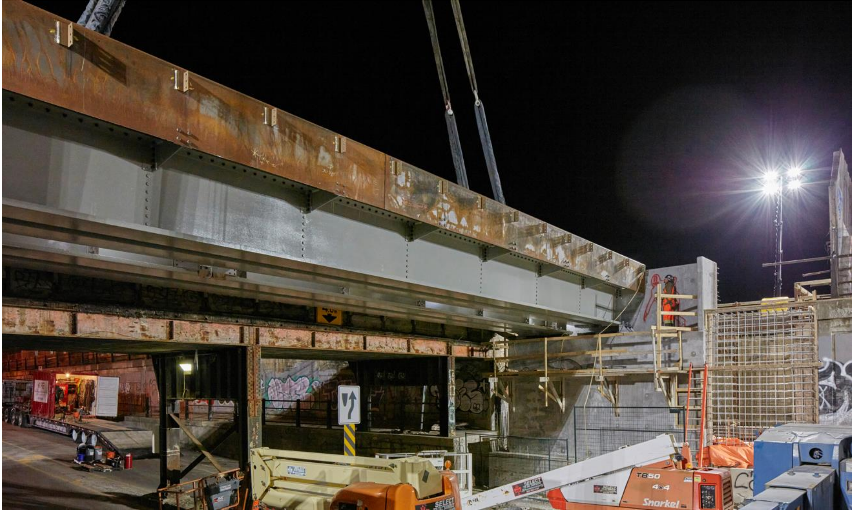
New steel girder on West Bloor Street Bridge.
