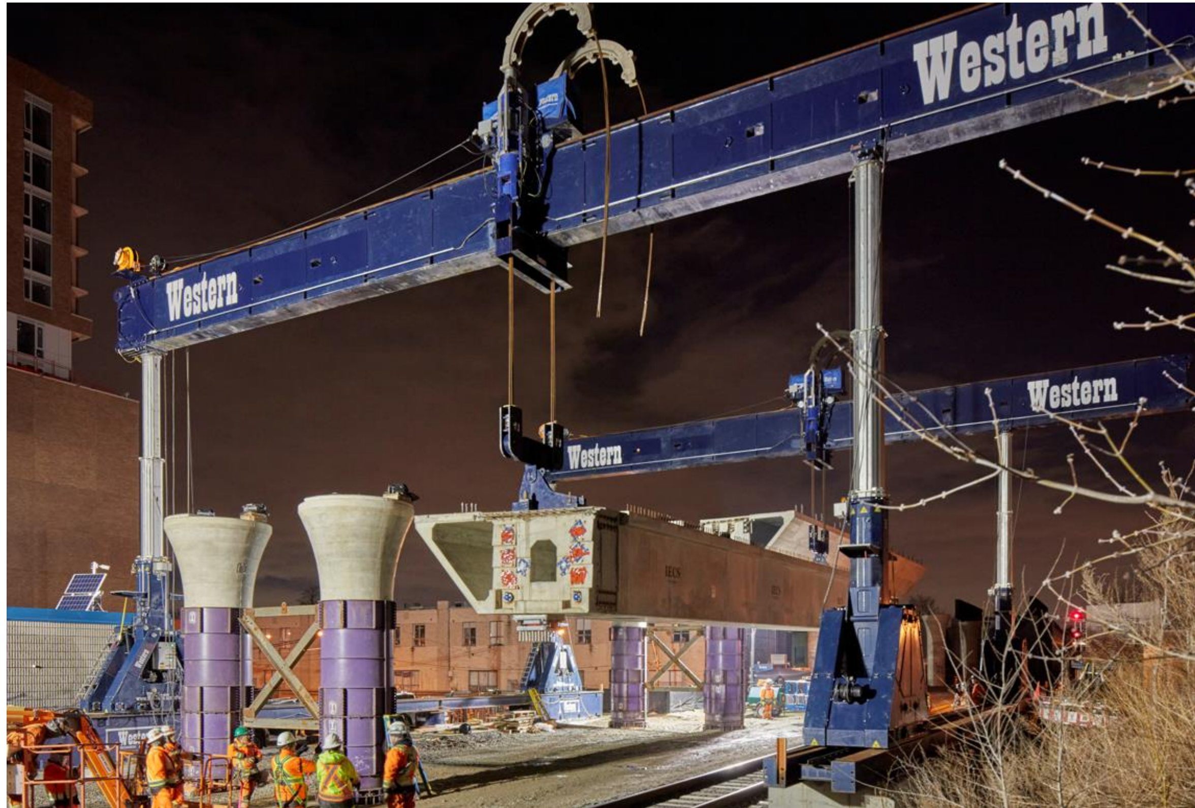
Gantry crane lifting girder over Dupont Bridge.
