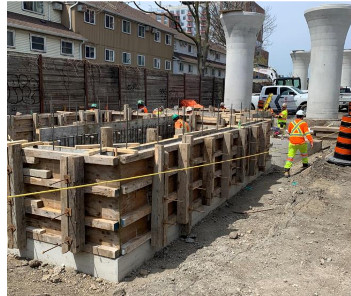
Formwork and rebar installation for Electrical and Communication Room footing walls.
