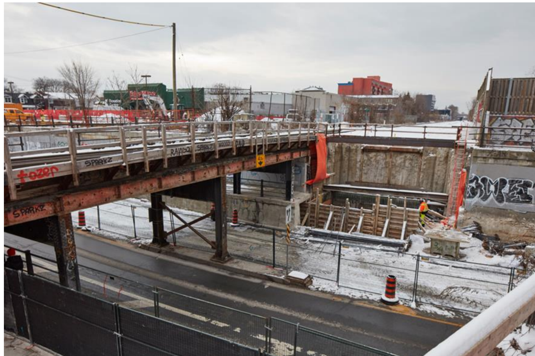
South bridge abutment construction (looking south).
