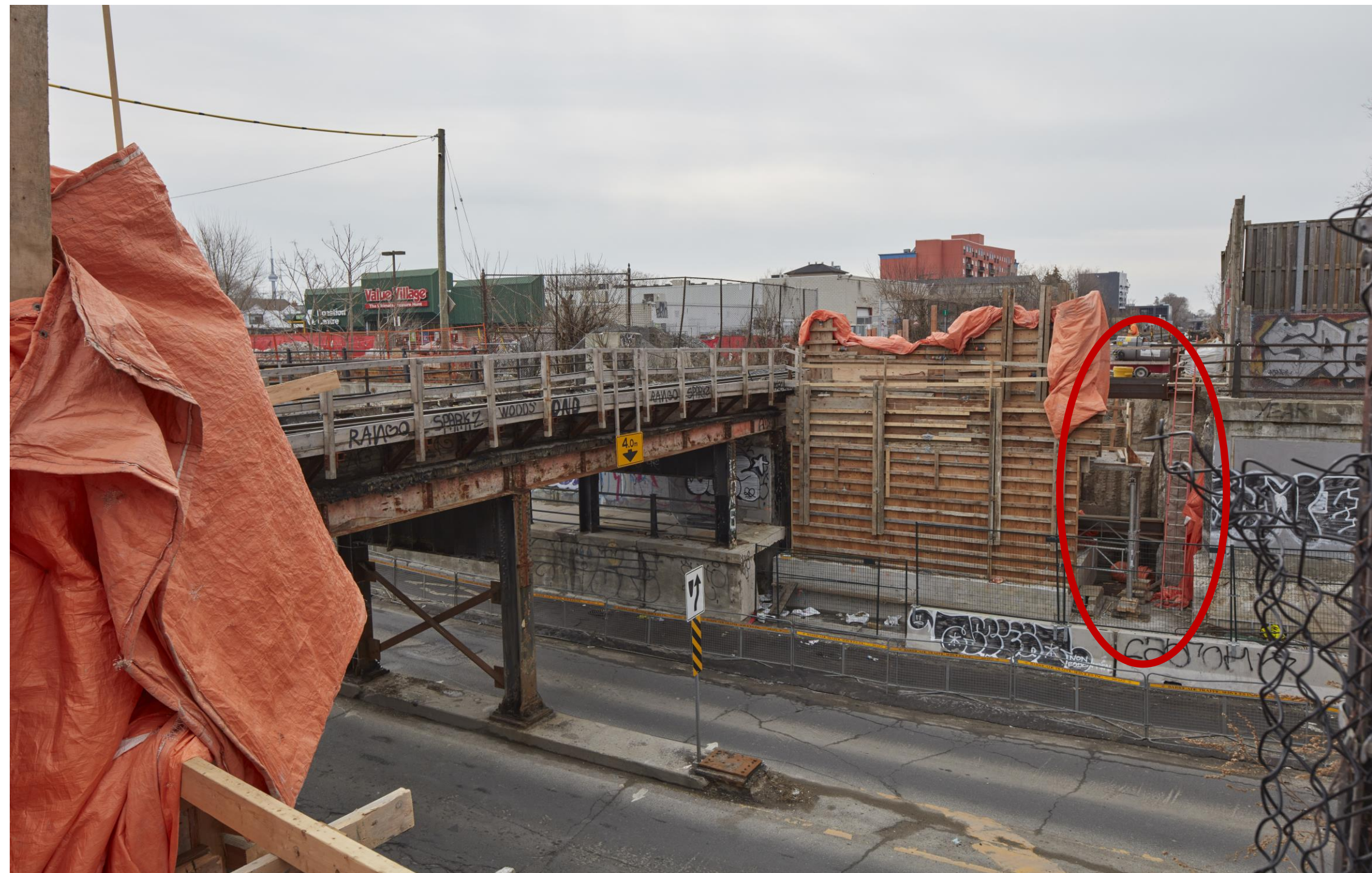
South bridge abutment and future retaining wall (looking south).
