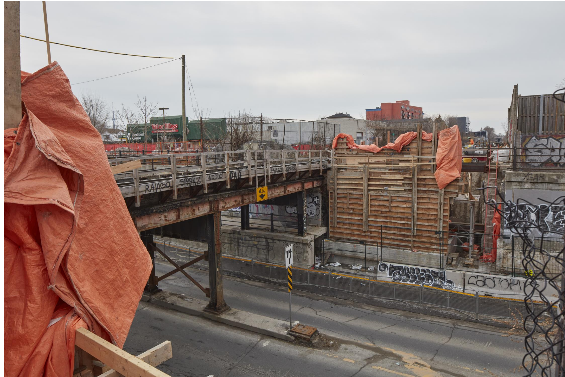
South bridge abutment prior to formwork removal (looking south).
