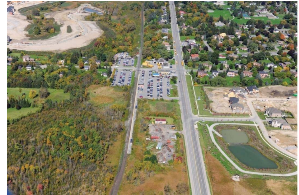
Photo 2-5: King City GO Station aerial image
