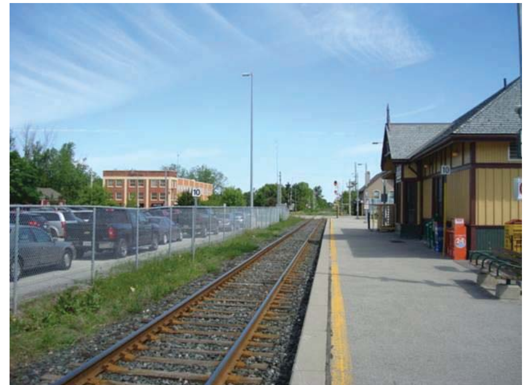
Photo 2-8: Aurora GO Station looking north - side platform
