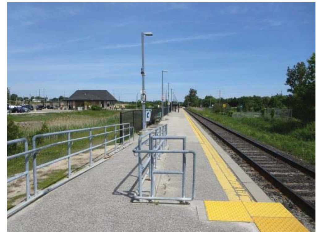
Photo 2-12: East Gwillimbury GO Station looking north - side platform
