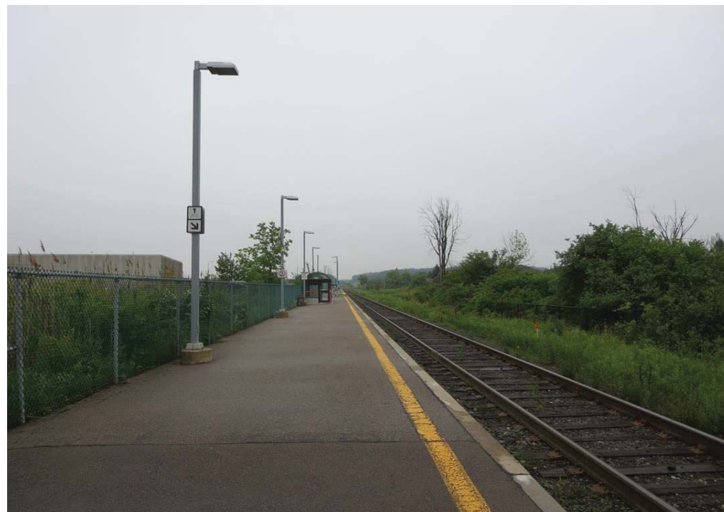
Photo 2-2: Rutherford GO Station looking north - side platform
