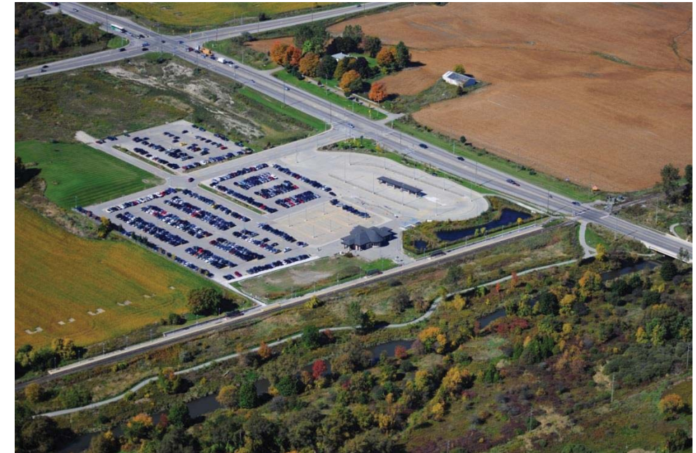
Photo 2-11: East Gwillimbury GO Station aerial image
