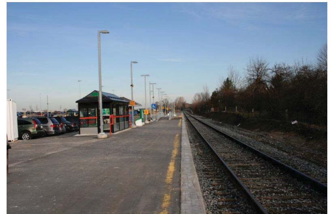
Photo 2-16: Barrie South GO Station looking north - side platform
