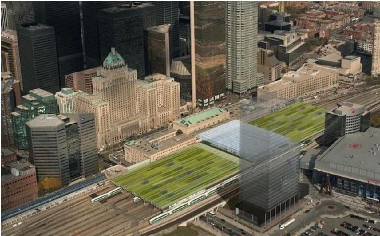
The central portion of the train shed roof will be replaced with a glass atrium. The train shed roof poses a constraint on the vertical clearance, and will require special design considerations for the implementation of the electrification system in the train shed area.
