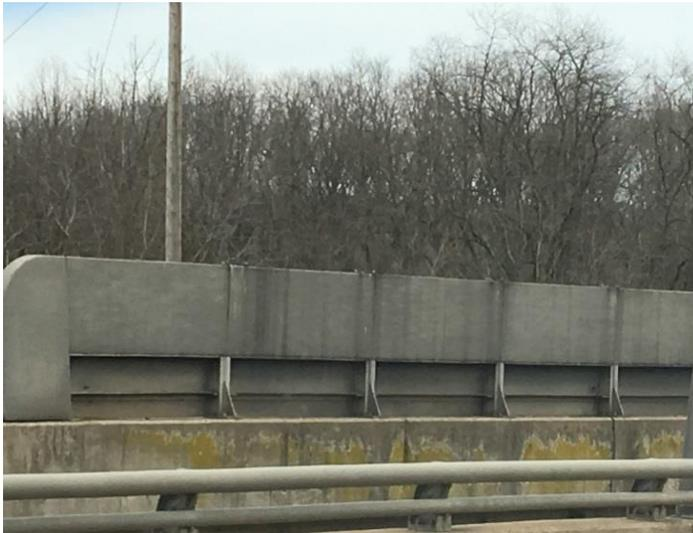
The length of the protection barrier will extend a minimum of approximately 3m laterally beyond the live parts of the overhead contact system, on either side the bridge. The barriers will be made of solid-faced material, and will be a minimum height of approximately 2m (barriers of greater heights may be required in areas where vandalism is prevalent). High voltage signage will also be provided as an additional safety measure.
