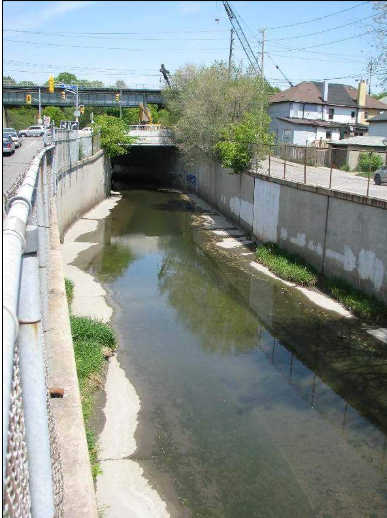
FIGURE 4-5 BLACK CREEK - DOWNSTREAM (SOUTH) OF RAIL CORRIDOR CROSSING, LOOKING UPSTREAM
