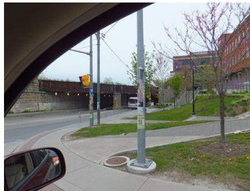
FIGURE 4-16 VIEW OF KING STREET SUBWAY LOOKING EAST
