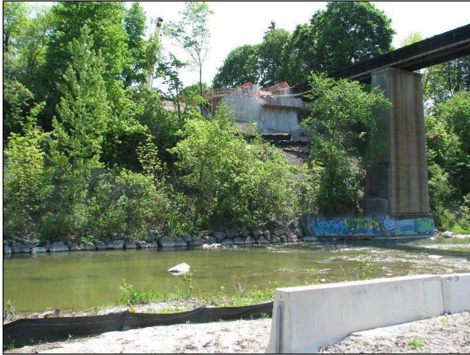
FIGURE 4-6 HUMBER RIVER - UPSTREAM (NORTH) OF RAIL CORRIDOR, LOOKING AT EAST BANK
