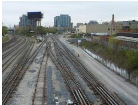
FIGURE 4-13 LOOKING WEST FROM BATHURST STREET BRIDGE.
