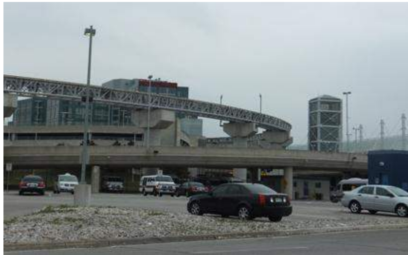
FIGURE 4-20 VIEW OF UP EXPRESS ELEVATED SPUR LINE TERMINATING AT TERMINAL 1
