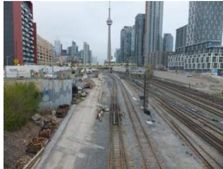
FIGURE 4-12 LOOKING EAST FROM BATHURST STREET BRIDGE
