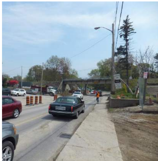
FIGURE 4-19 VIEW LOOKING SOUTH ALONG WESTON ROAD
