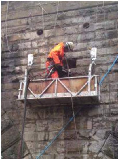
FIGURE 6-6 EXAMPLE OF ROPE ACCESS INSTALLATION METHOD
