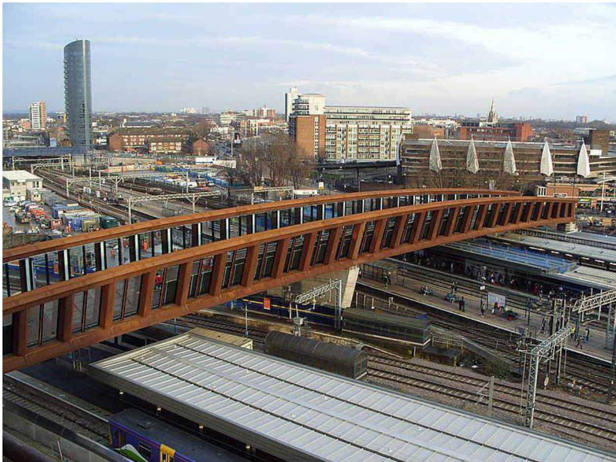
FIGURE 6-8 EXAMPLE OF BRIDGE PROTECTION BARRIER
