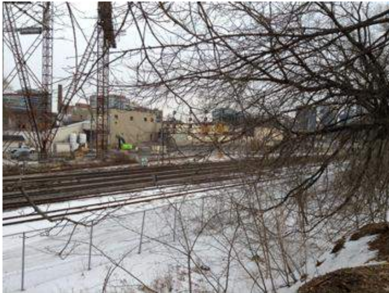
FIGURE 6-16 VIEW LOOKING NORTH FROM GARRISON COMMON OF THE LAKESHORE LINE AND ORDNANCE TRIANGLE AND THE PROPOSED PARALLELING STATION LOCATION.
