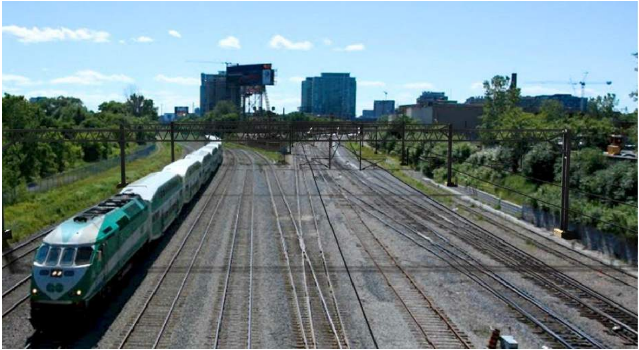
FIGURE 6-15 CORRIDOR AS VIEWED WEST OF BATHURST STREET BRIDGE
